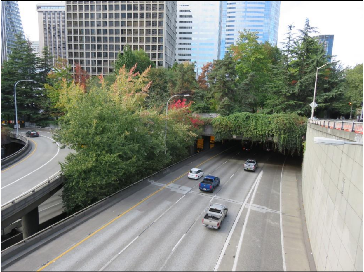
Photo 1. Freeway Park's Great Box Garden over I-5, view north.
