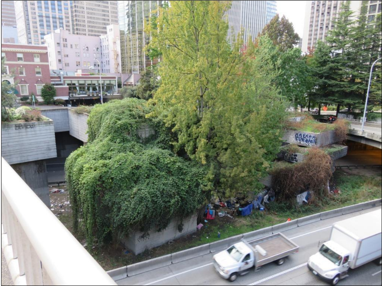
Photo 2. Freeway Park's Great Box Garden over I-5, view northwest.
