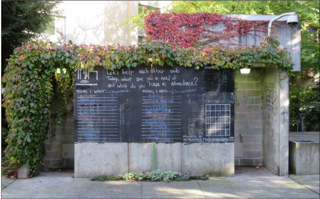
Photo 16. Freeway Park comfort station with elevator to the excluded Freeway Park Garage to the rear, view east.
