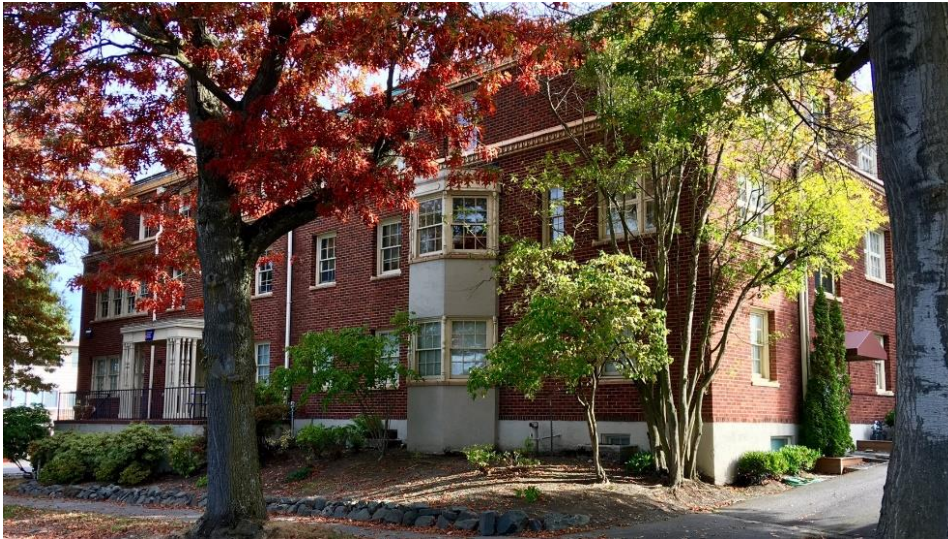
Front (West face) of Subject
