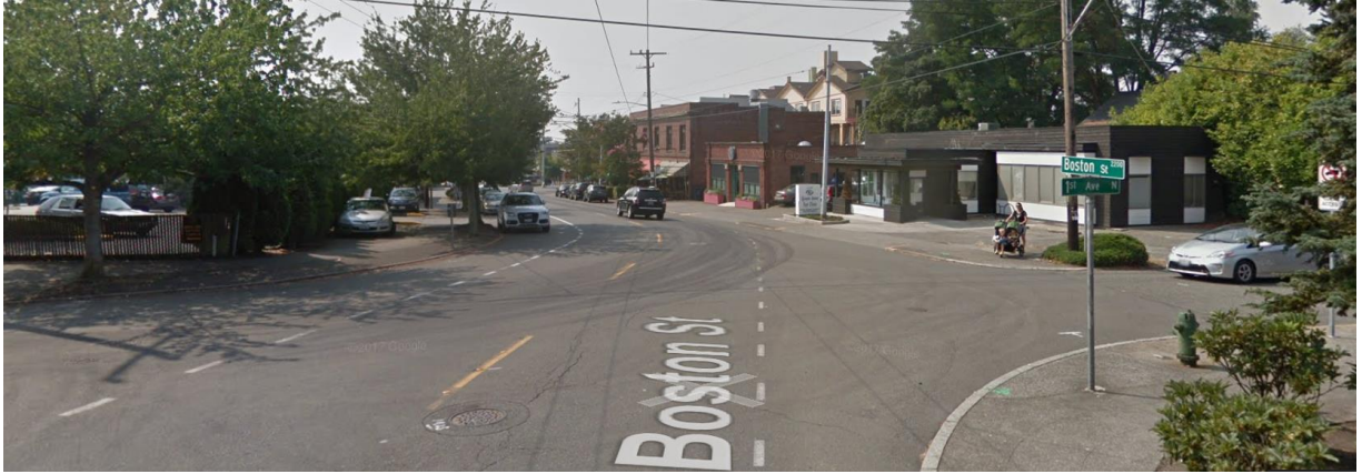
Commercial Buildings NW of Subject
