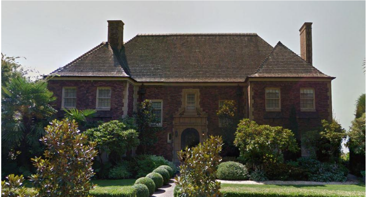
HISTORIC STUART-BALCOM HOUSE – 619 W. Comstock Street (a designated landmark)
