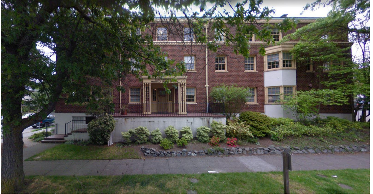
Front Side (West face) - May 2008
