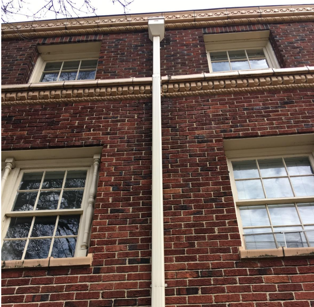
Detail of Windows, fascia and rain leader on front of Subject
