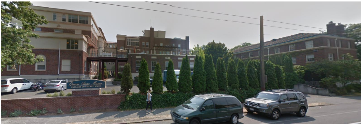
Queen Anne Manor on South Side of Boston St. – Subject is seen on the right.
