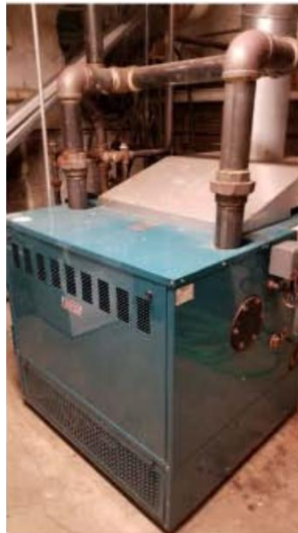
Boiler Room in Basement
