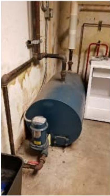
Boiler Room in Basement
