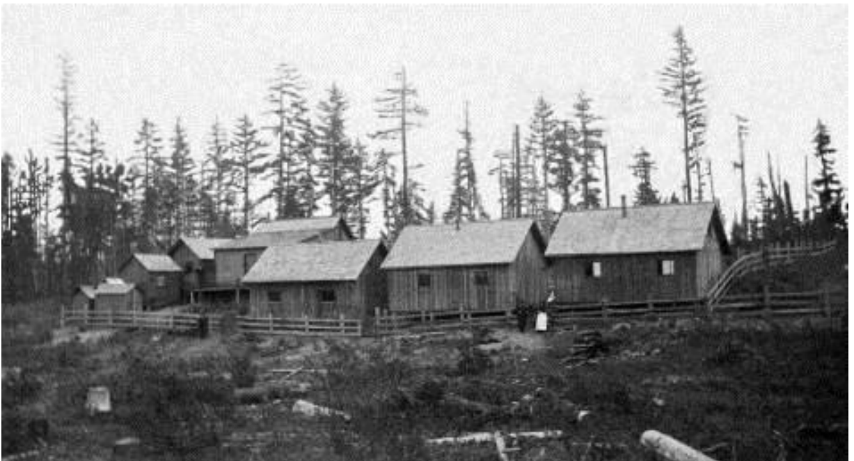
Original top-of-Queen Anne settlement, 1889 – See: Setting: Immediate Neighborhood and History above.
