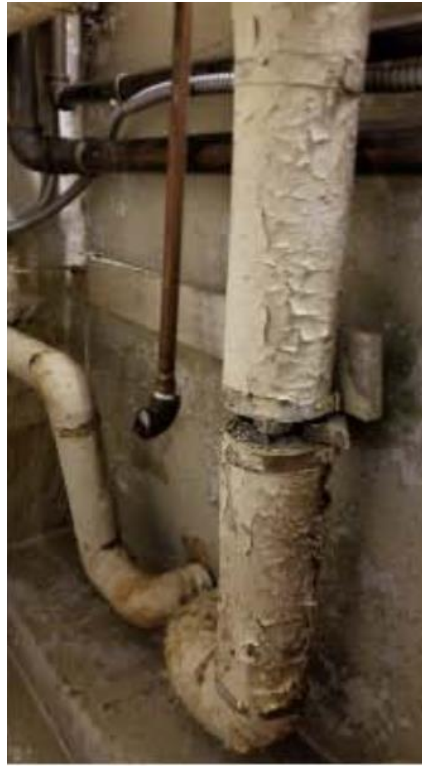
Boiler Room in Basement
