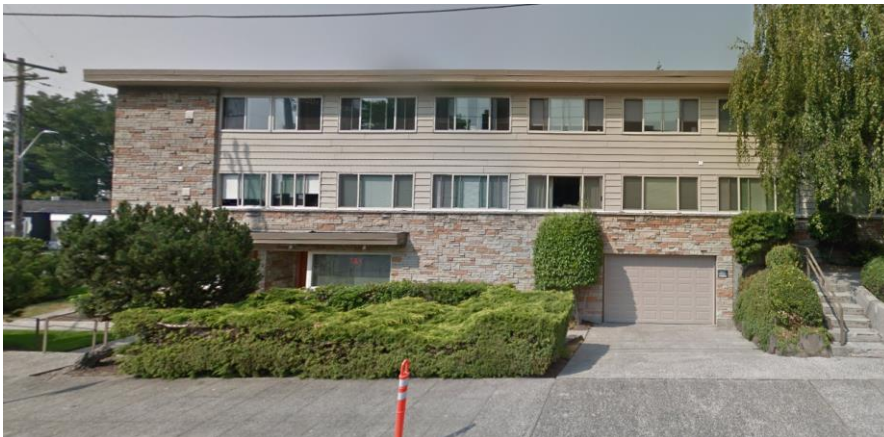
Apartment Building Directly Across Boston St. – North from Subject
