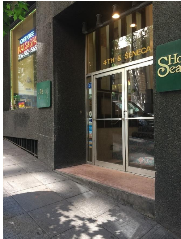
Figures 54 & 55. Above left, the south entry to the retail space at 317 Seneca Street. Above right, the main entry to the hotel lobby. The recessed, aluminum framed storefront entries, sidelights, transoms, and infill date from the 1960s.
