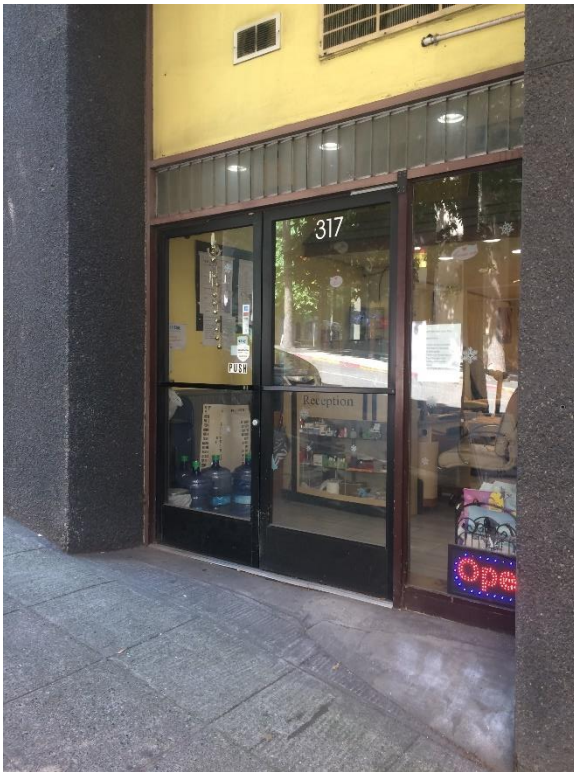
Figures 54 & 55. Above left, the south entry to the retail space at 317 Seneca Street. Above right, the main entry to the hotel lobby. The recessed, aluminum framed storefront entries, sidelights, transoms, and infill date from the 1960s.
