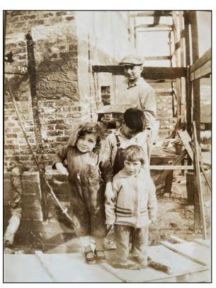
Fig. 71 – (Four photos) Ca. late 1920s-early 1930s masonry construction, showing Fausto on his home-made scaffolding with several of his children. Fausto received a building permit in 1928, but may have begun work at the site as early as 1926. We know the stuccoing was complete by 1937. Note the continuous concrete lintel serving as header for windows and doors. (VC)
