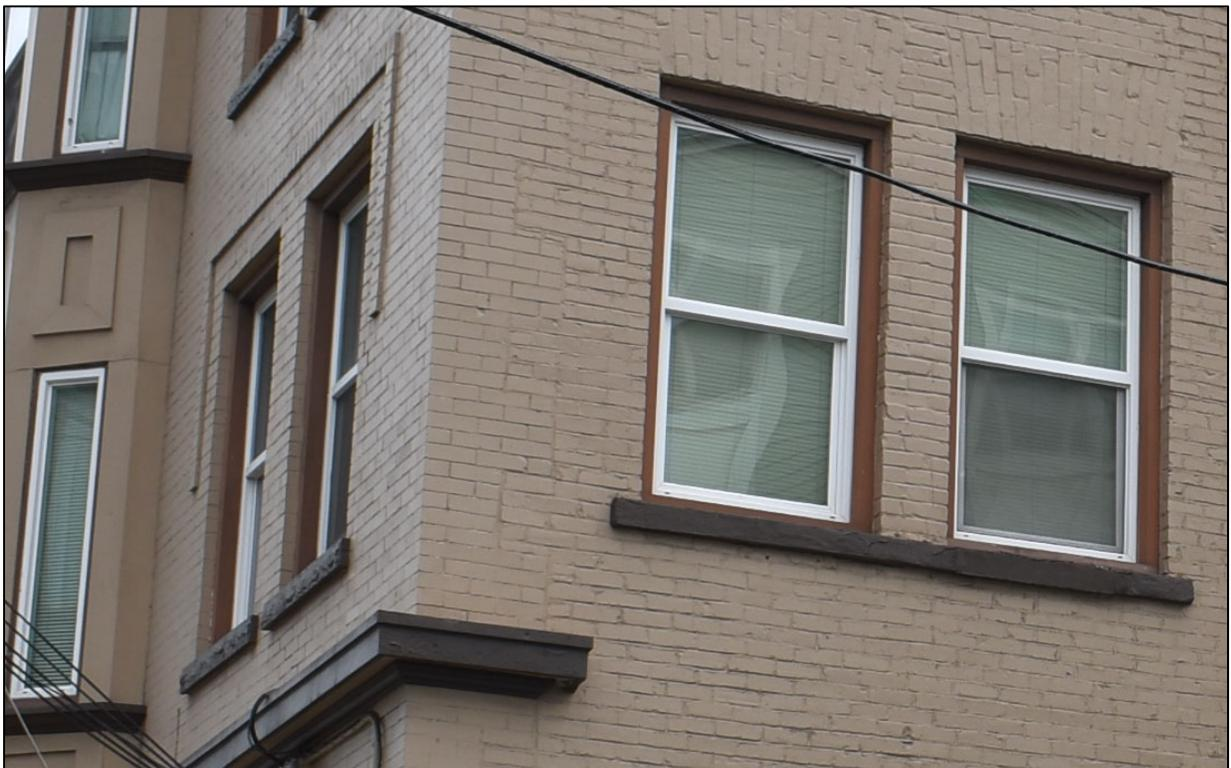
Fig. 22 – North and west facades, detail showing face brick meeting common brick at building corner.
