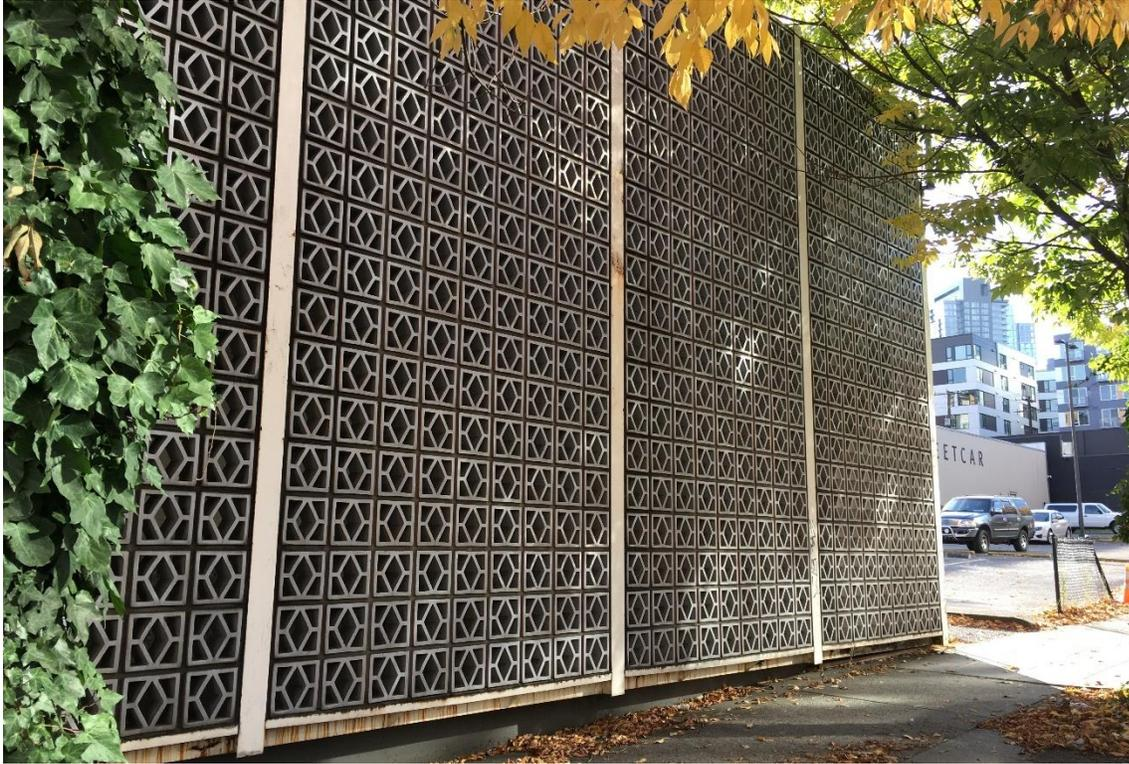
**FIGURE 9: WEST ELEVATION, DETAIL SHOWING TERRACOTTA TILE SOLAR SCREEN (2017)**
