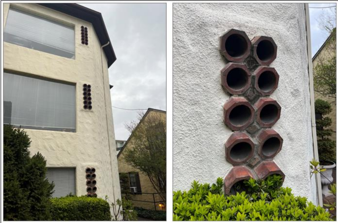
Figure 92: Anhalt Apartments – Windows and Ventilation Tubes (Camera facing North)
