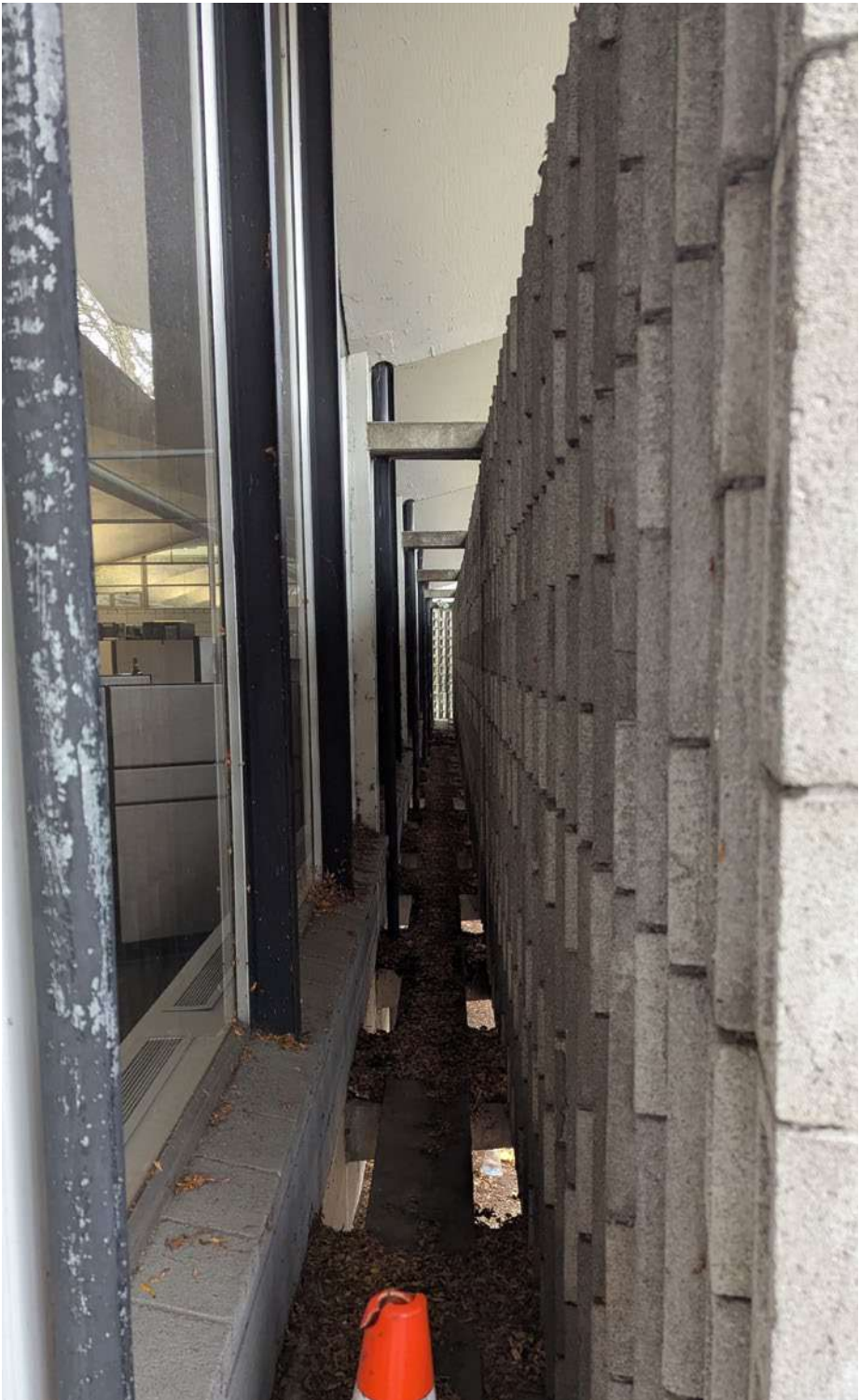
BLOCK WALL SEPARATION FROM BUILDING
