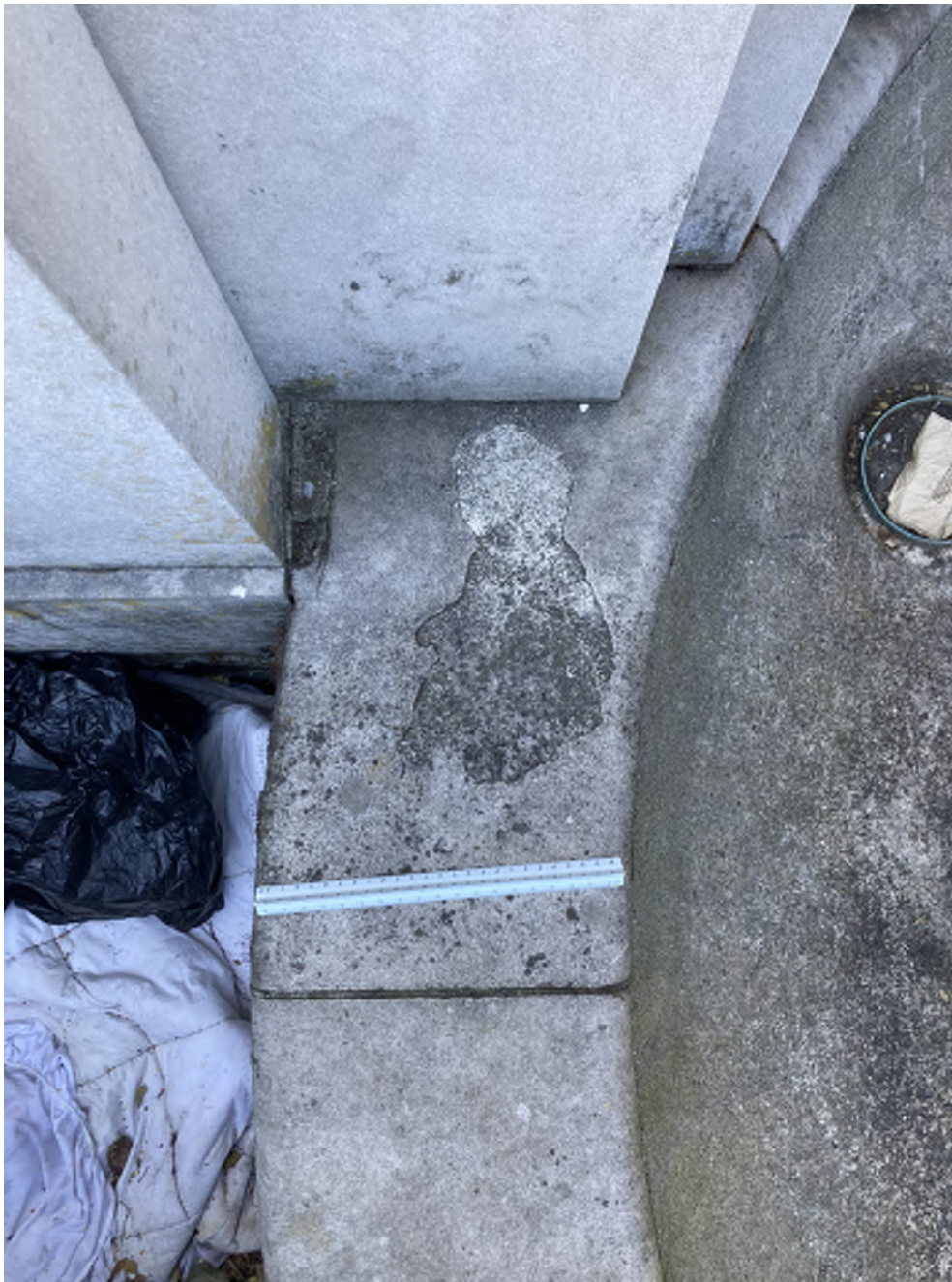
South Fountain Basin Edge - Stone Deterioration
