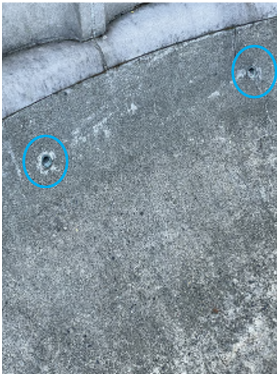
Water Overflow Pipes at Rim
