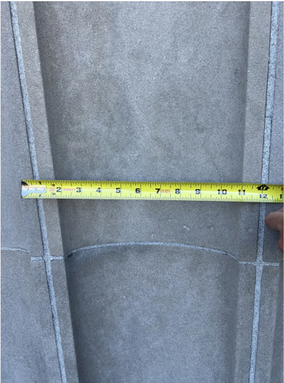
Fountain Backdrop Fluting - Jointing and Stone Condition
