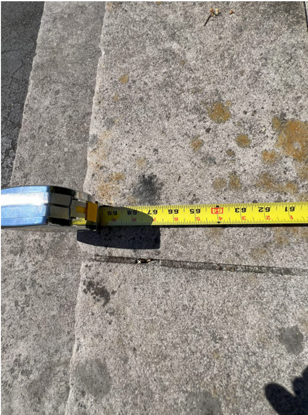
Memorial Steps - Stone Joint, Discoloration, and Moss
