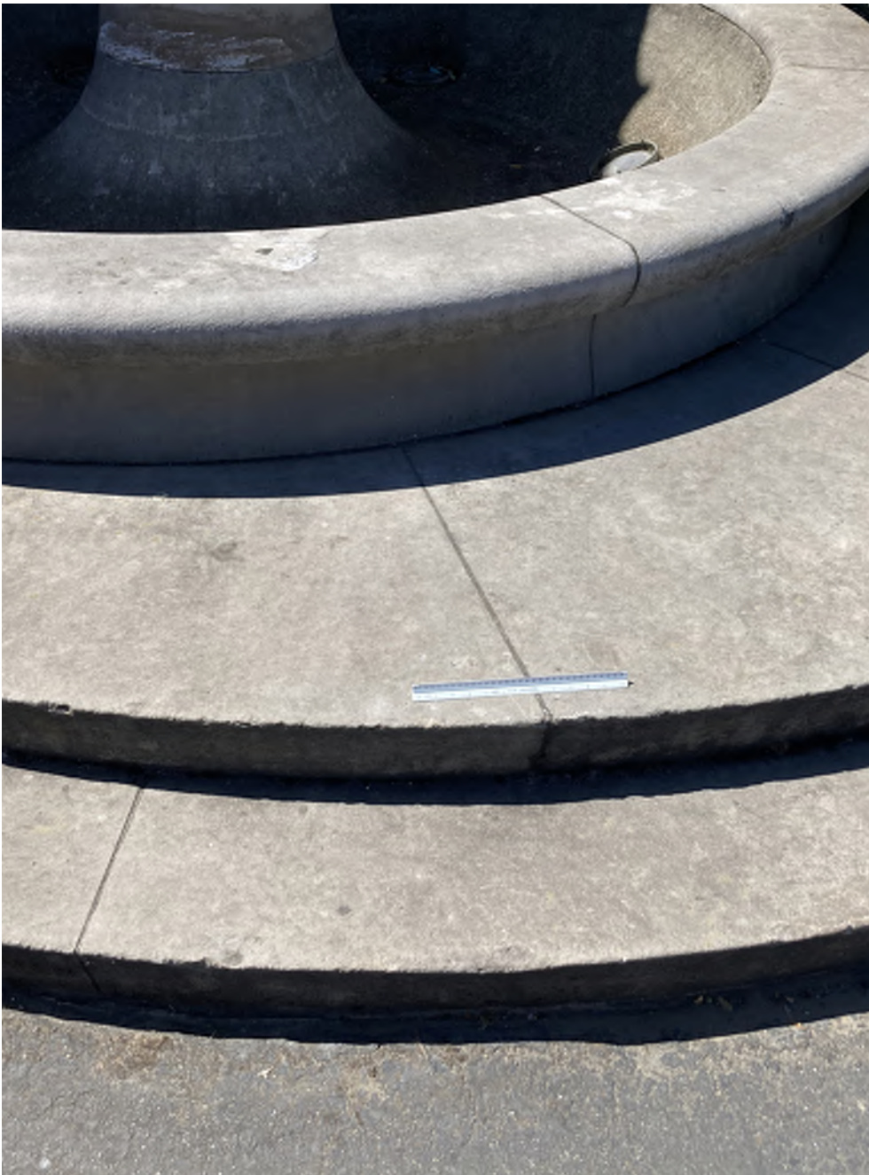
South Basin Steps - Nosing Chips and Discoloration
