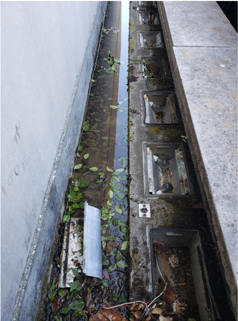
Memorial Wall Lighting Trench - Fixture Condition + Standing Water
