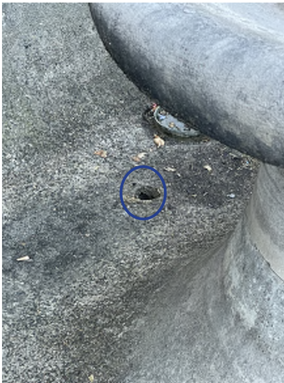
Water Outlet at Basin Low Point
