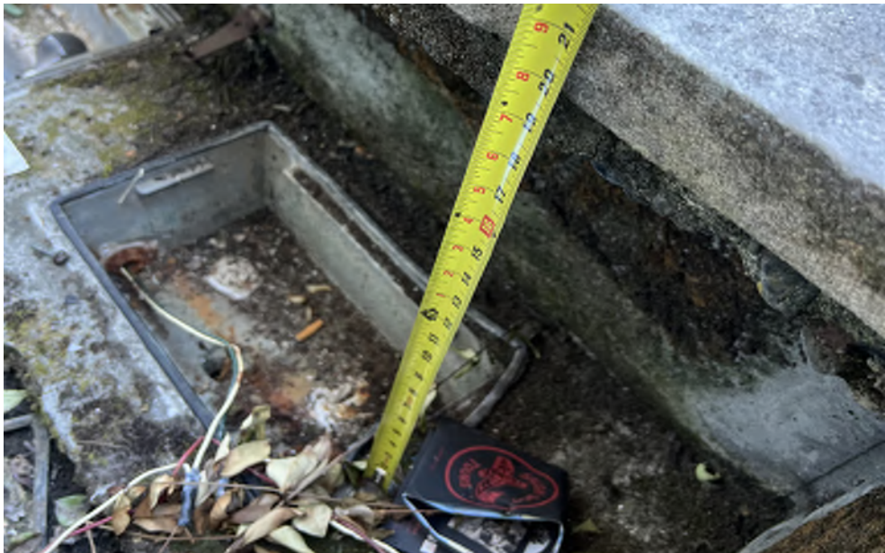
Memorial Wall Light - Fixture Housing and Wiring Condition
