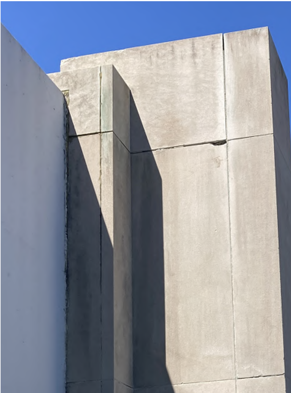
North Memorial Stone Wall and Stadium Concrete Wall at Top of Walls - Stone Chips at Jointing
