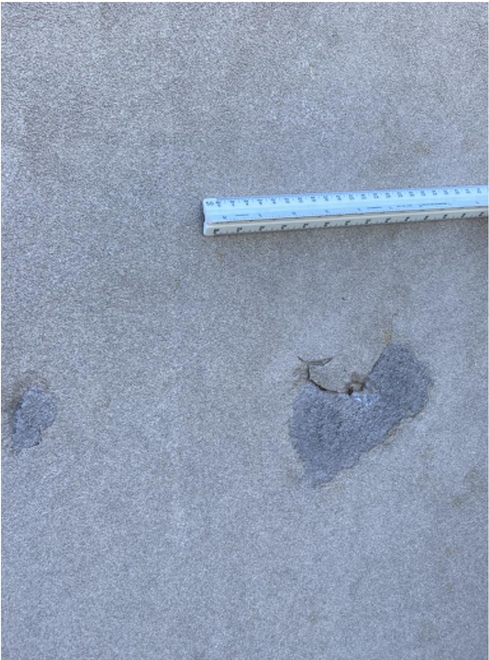
Memorial Wall - Stone Patch Work, Two of Three
