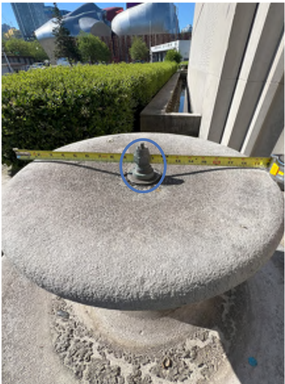
Water Inlet at Pedestal Top
