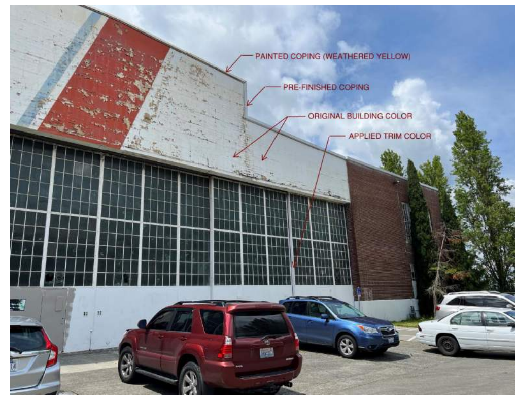
6 ROOF EDGE EAST D5.2a 1" = 1'-0"
