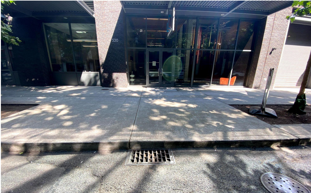
Storm drain looking east
