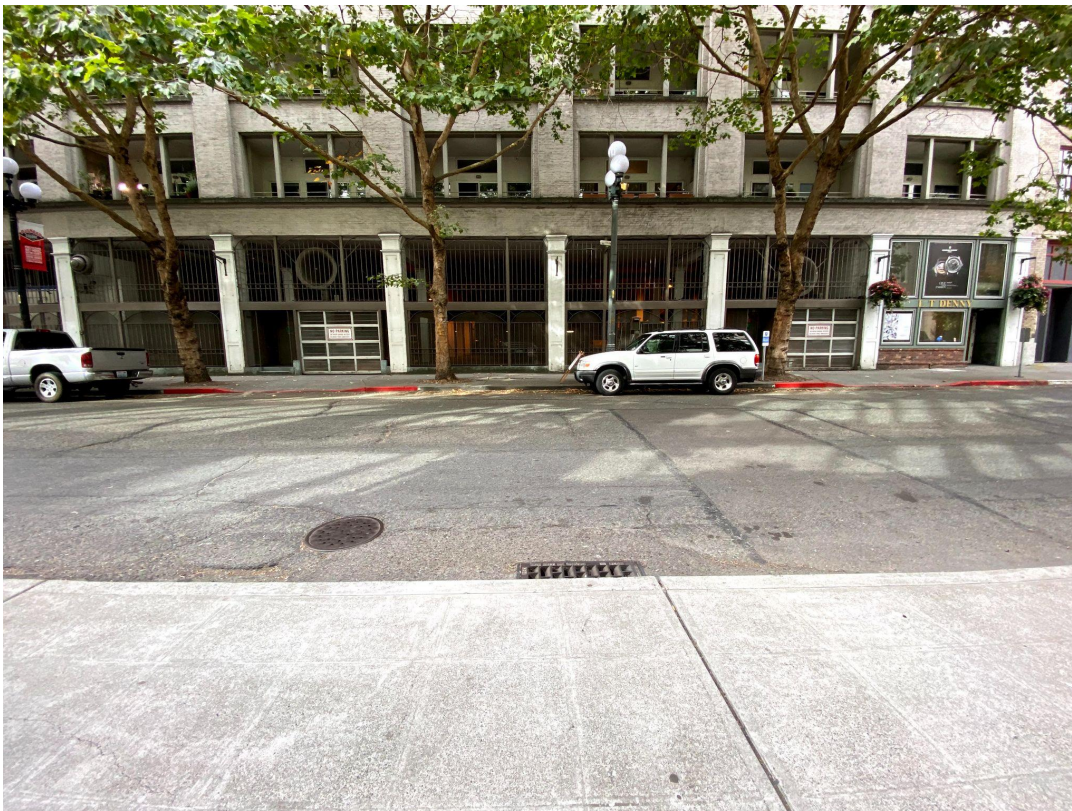
Storm drain looking west
