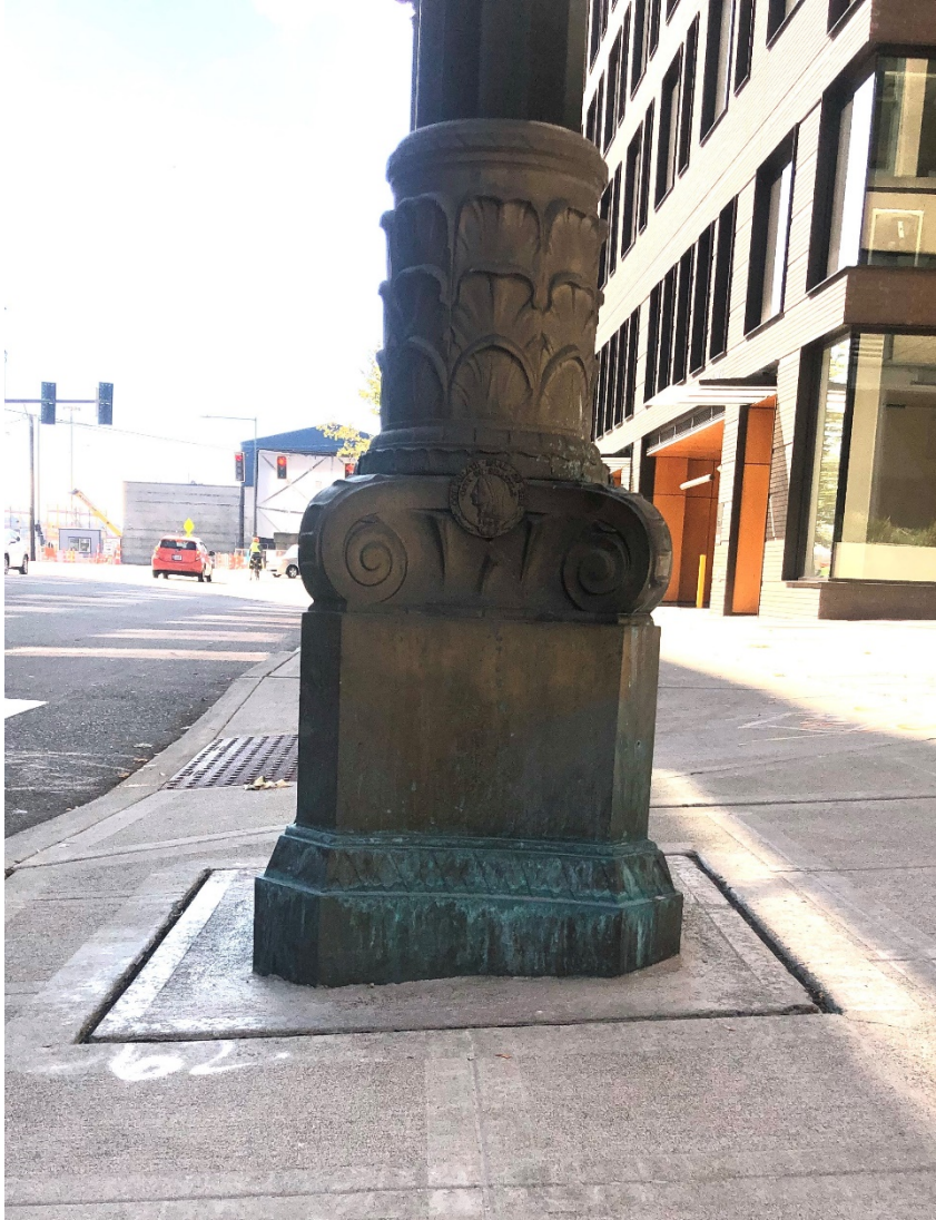
Base Installed in 2019
