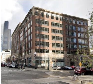
Figure xxx. A building that features a top middle and base façade composition. Note the light-colored masonry storefront (base), the repetitive window patterns of the second through sixth stories (middle, and unique design of the top story (top).
