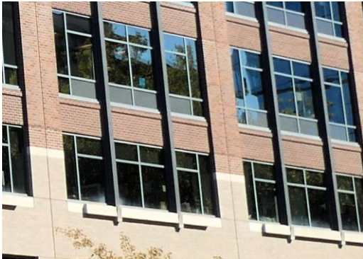
Figure xxx. This contemporary Pioneer Square building features windows with multiple panes and extended sills which add scale and nuanced detailing. Additionally, the groups of windows are recessed from the pilasters to enhance the façade’s sculptural qualities and visual “rhythm”.
