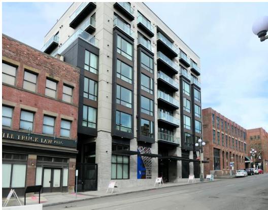
Figure xxx Building as viewed as part of a block front.
