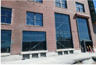
Figure xxx. The Alaskan Way facade of this building has been altered in an appropriate manner to accommodate new uses.
