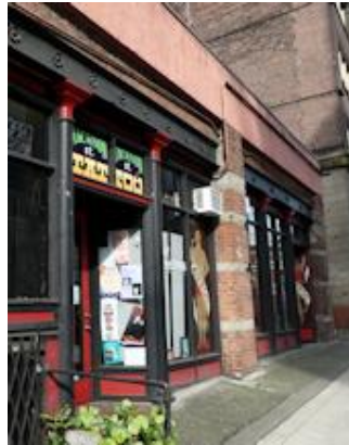
Figure xxx. Some buildings feature cast iron elements.
