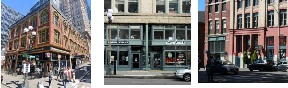
Figure xxx. Four examples of appropriate color palettes for Pioneer Square: Natural materials (brick and stone), complementary trim, and brighter colors reserved for accents and signs. Note the subtle but effective two-color scheme of the Jimmy John's/Evergreen storefronts.
