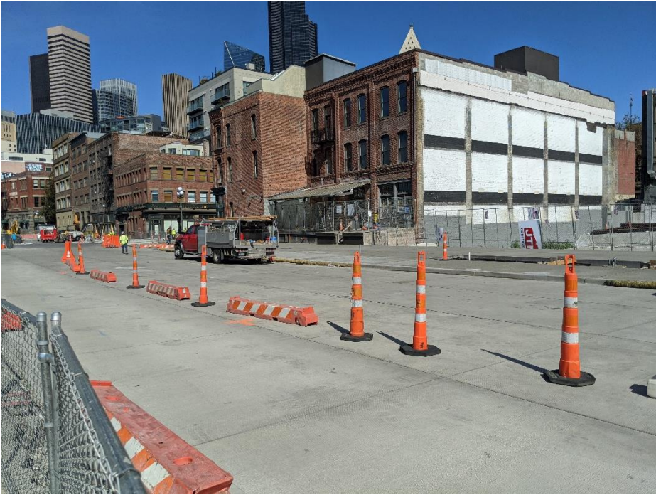
NB Jackson Street Station
