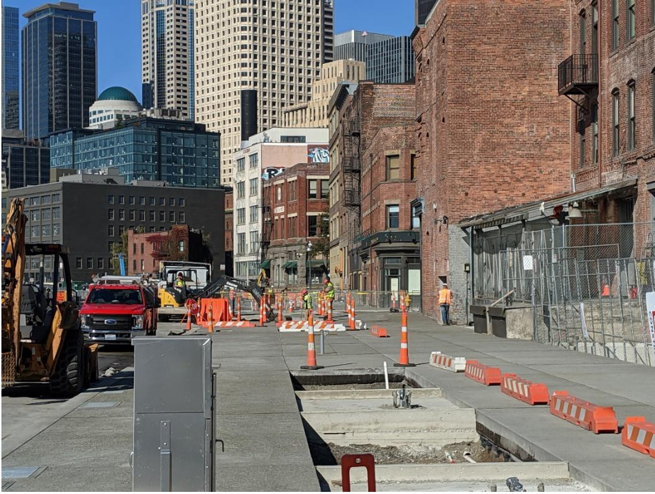
NB Jackson Street Station
