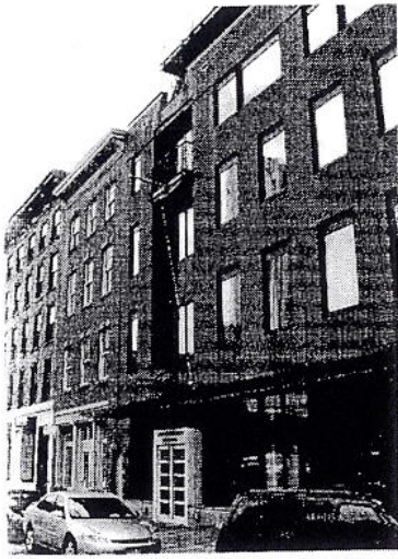
Figure 5. Seamen's Church Institute, South Street Seaport Historic District, New York, N.Y. James Stewart Polshek and Partners, 1992. Photo by Steven Semes.
