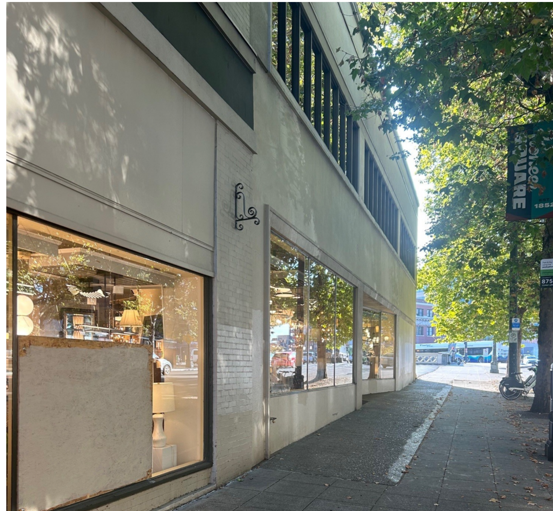
PHOTO #1 - 210 2nd Ave Ext. S. - Looking S.E.
