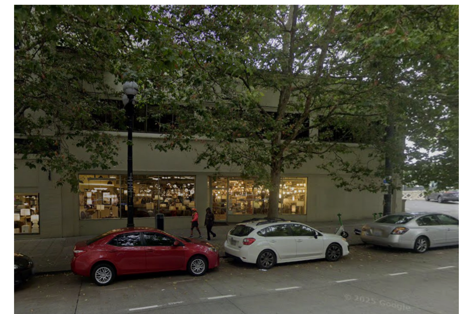
PHOTO #6 210 2nd Ave Ext. S. - Looking E. August 2025 Google Street View
