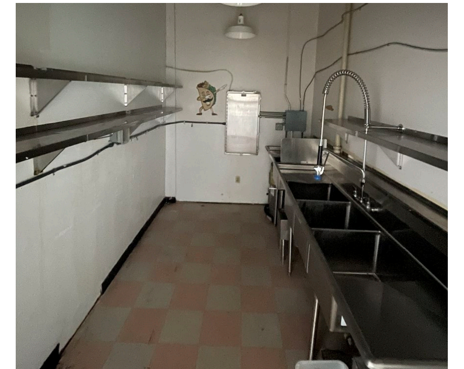
East Wall Kitchen
