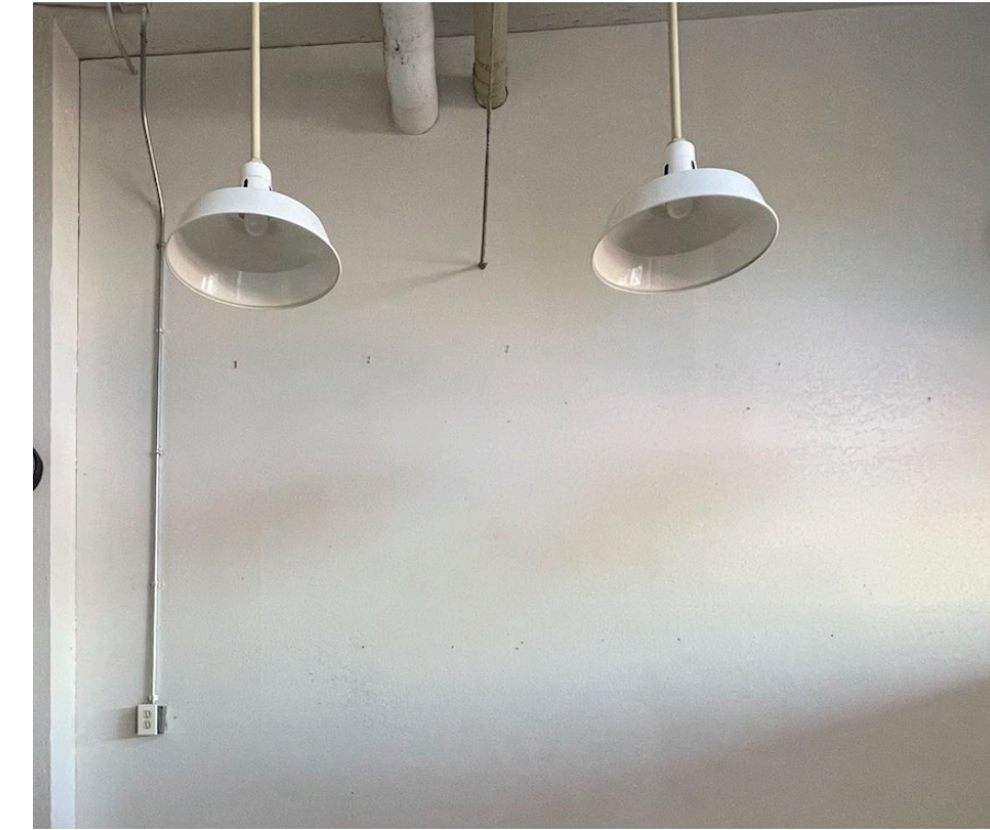
Keeping existing light fixtures
