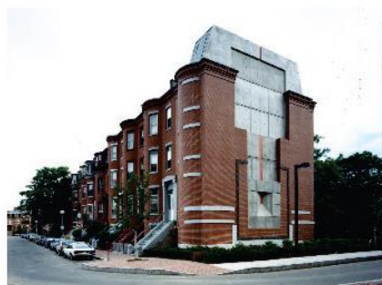
這個波士頓的例子將通風設施與歷史建築結合 This example in Boston illustrates an example of integrating ventilation with historic building
