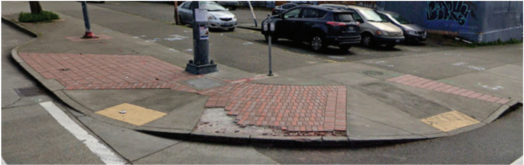
EXISTING CONDITION OF BRICK PAVING AT CORNER
