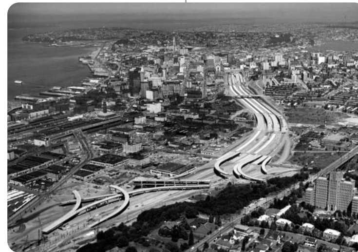
CONSTRUCTION OF I-5 SPLITS THE CHINATOWN INTERNATIONAL DISTRICT IN TWO AND DISPLACES 15 CITY BLOCKS OF RESIDENTS AND RETAIL
