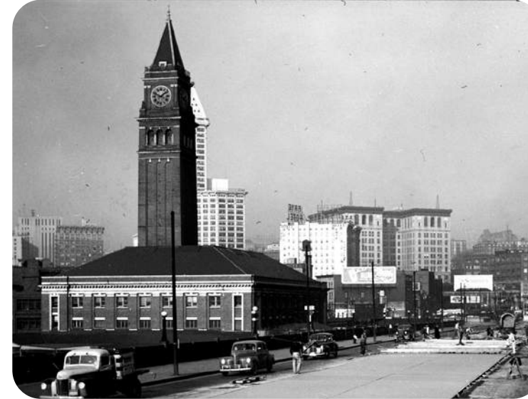
KING STREET STATION COMPLETED
