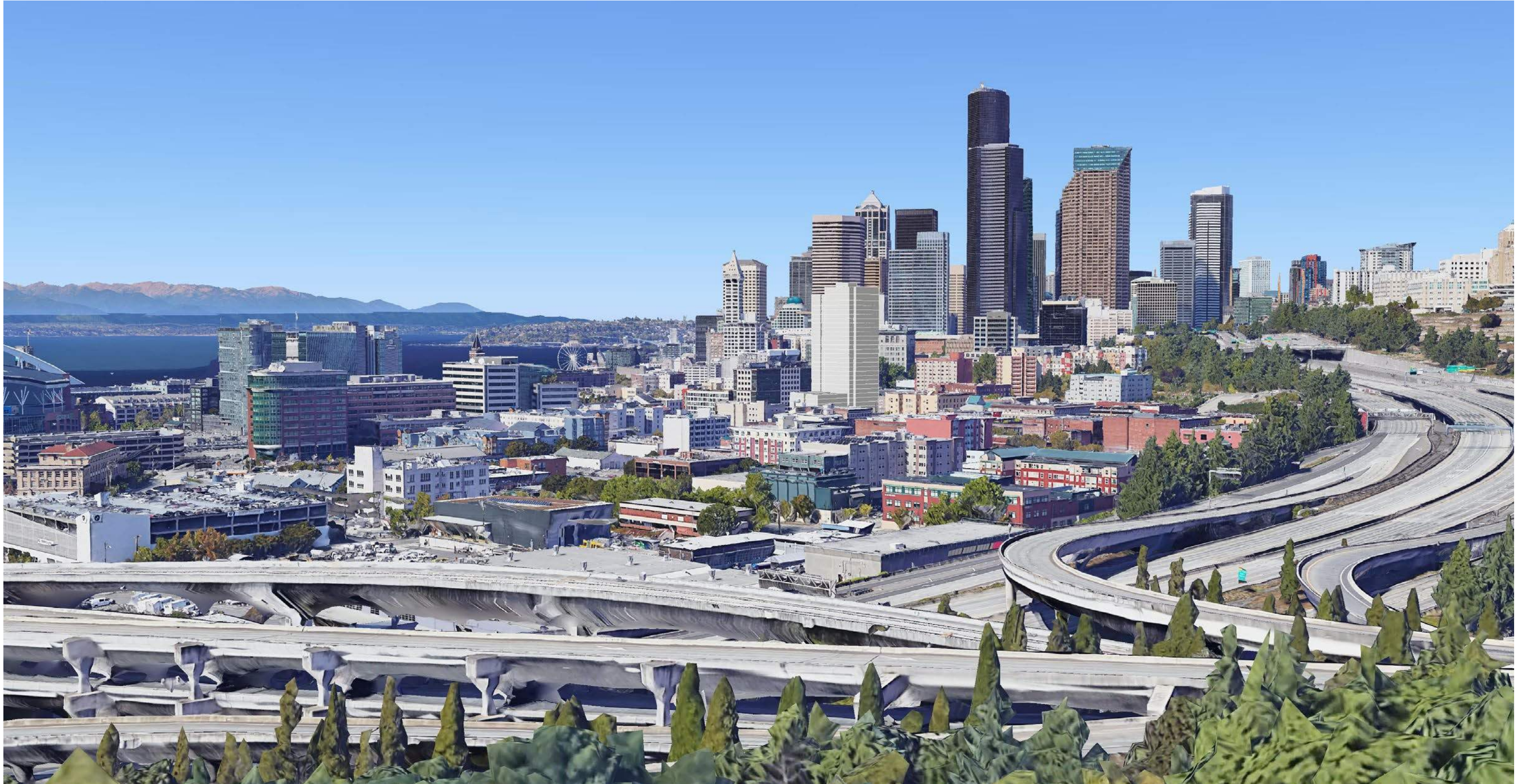
View from 12th Ave. overpass looking northwest towards the project.
