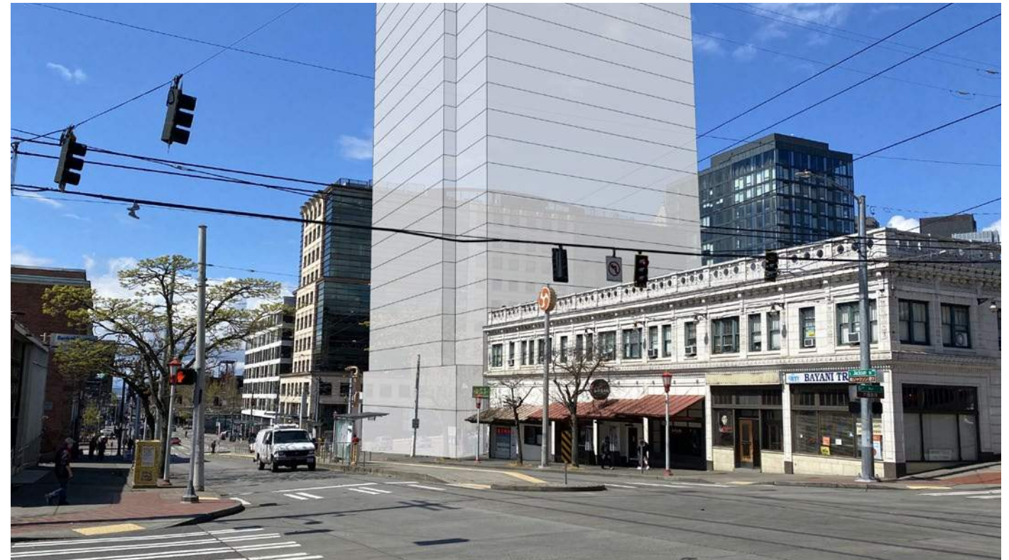
View of the project from South Jackson looking west near 6th. Ave
