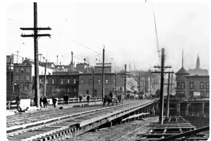
JACKSON STREET REGRADE COMPLETED
