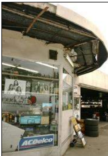
Below, views in 2008 of the Service Station (Building A in the King County Assessor’s records). Some of the steel framing, cladding and steel framed windows were visible at that time, along with the “top-hat” style overhang.
