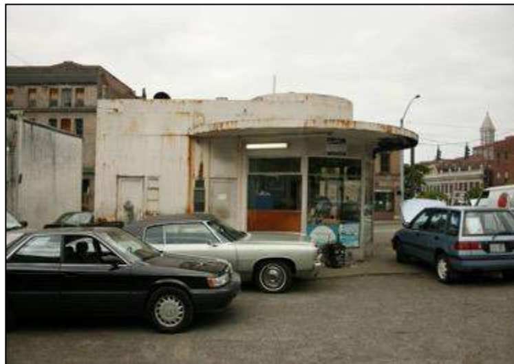
Below, views in 2008 of the Service Station (Building A in the King County Assessor’s records). Some of the steel framing, cladding and steel framed windows were visible at that time, along with the “top-hat” style overhang.
