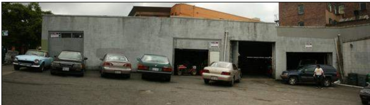
Below, views in 2008 of the Service Station (Building A in the King County Assessor’s records). Some of the steel framing, cladding and steel framed windows were visible at that time, along with the “top-hat” style overhang.
