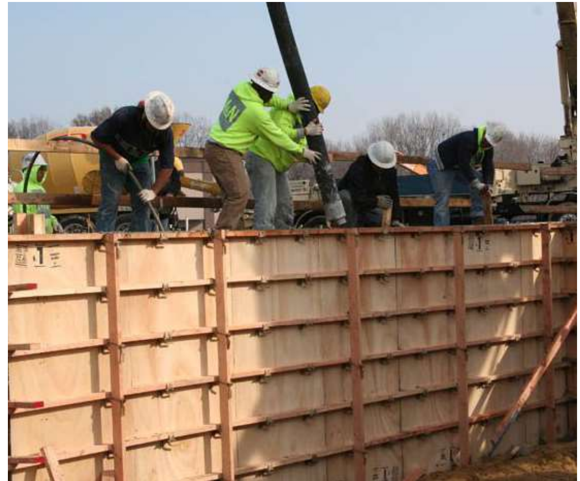
POURING CONCRETE BACKING WALL
