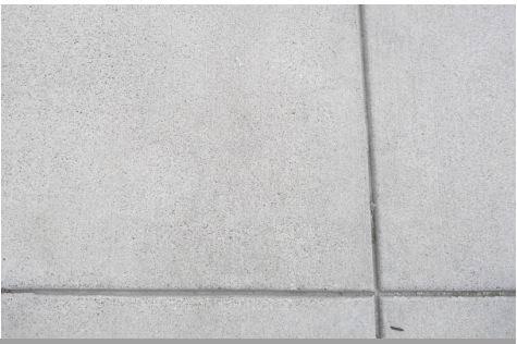
NATURAL CIP CONCRETE SIDEWALK, STANDARD COS 2' X 2' SCORING
