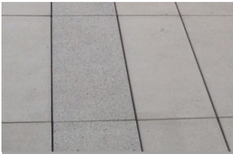
INTEGRAL COLOR CIP CONCRETE PAVING, 1' VERTICAL SCORING
