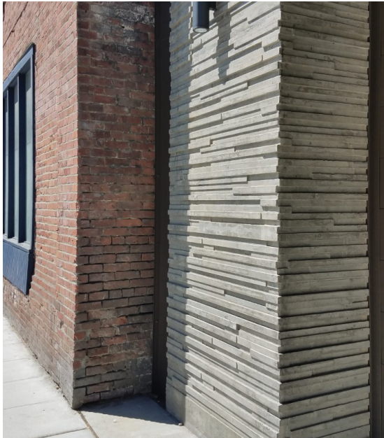
CONCRETE WALL W/ SPECIALTY FORMWORK AT EXT. PASSAGEWAY ENTRY
