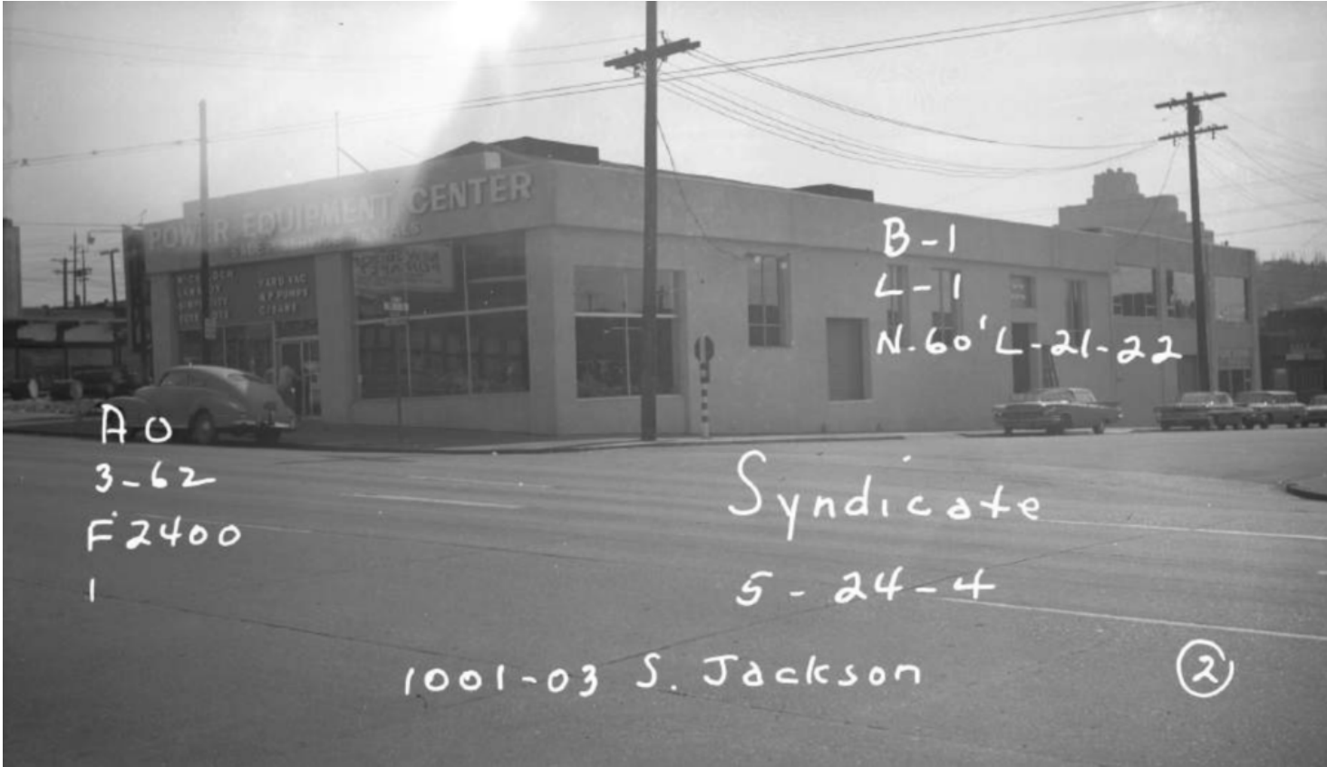
A 1962 VIEW LOOKING SOUTHEAST AT THE NORTH AND WEST FACADES OF 1001 S. JACKSON AND THE WEST FACADE OF 410 10TH AVE S., FOLLOWING BUILDING ALTERATIONS. AT THIS POINT THE BUILDINGS WERE CONSOLIDATED AS ONE TAX PARCEL AND "UNIFIED" VISUALLY BY A SINGLE ARCHITECTURAL TREATMENT. (KING COUNTY TAX ASSESSOR PROPERTY RECORD, PUGET SOUND REGIONAL ARCHIVES)
