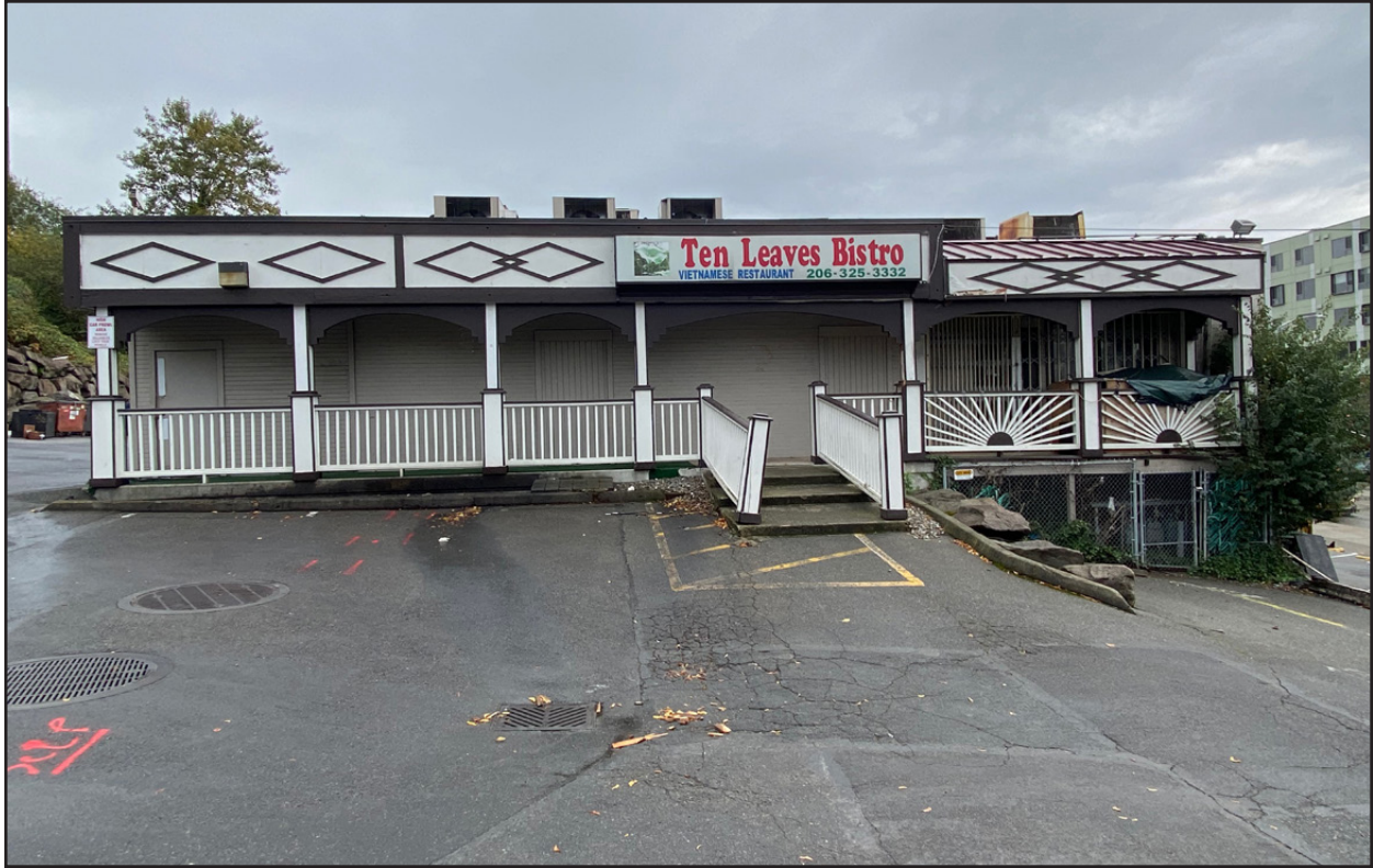
Figure 17 • Building 1, eastern facade
