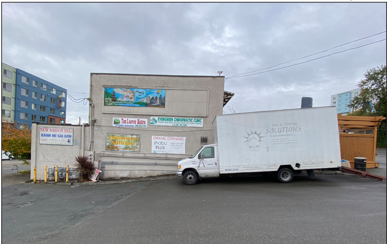
Figure 24 • Building 2 eastern facade
