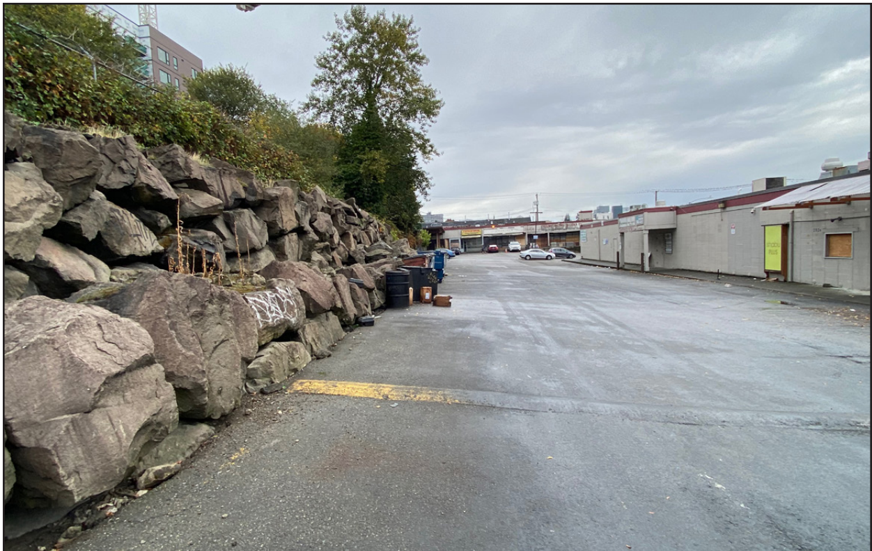
Figure 9 • Northern side of subject site
