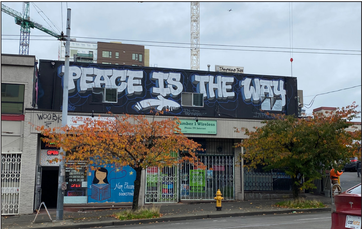
Figure 22 • Building 2 southern facade
