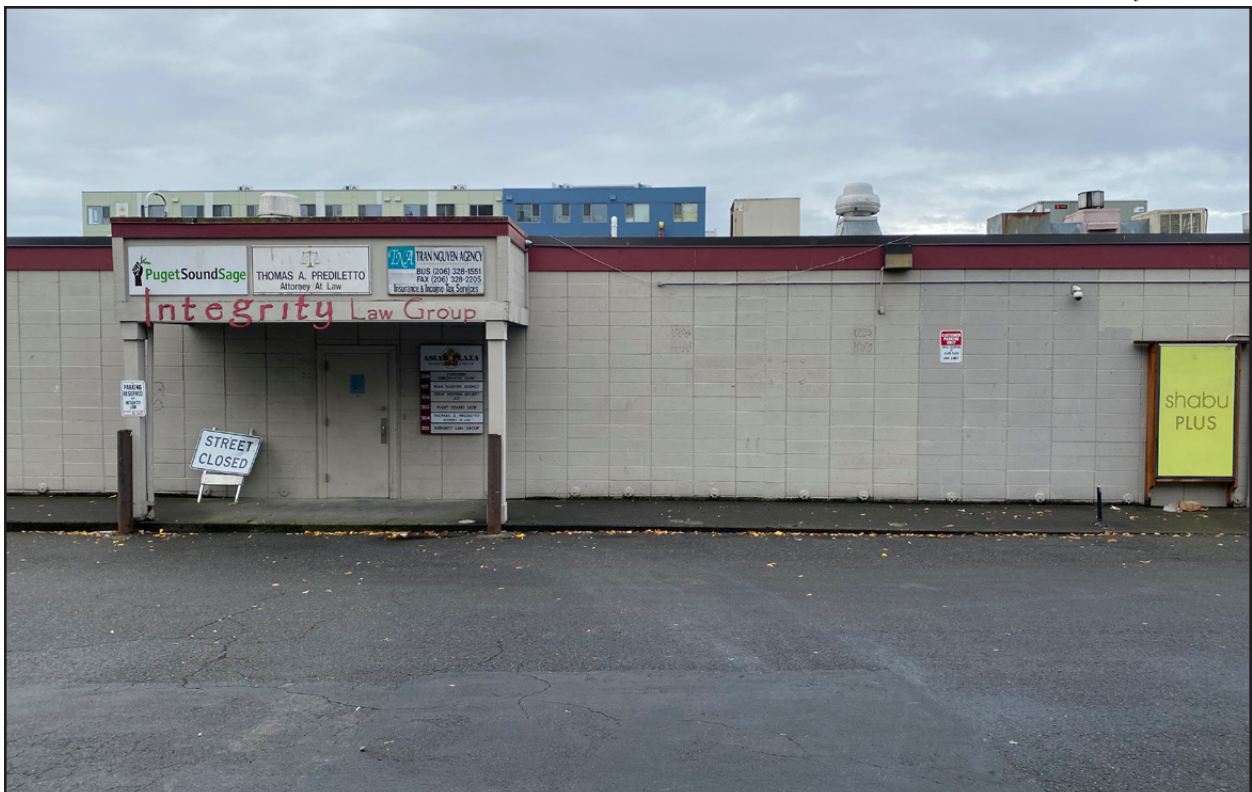
Figure 20 • detail of northern facade building 1
