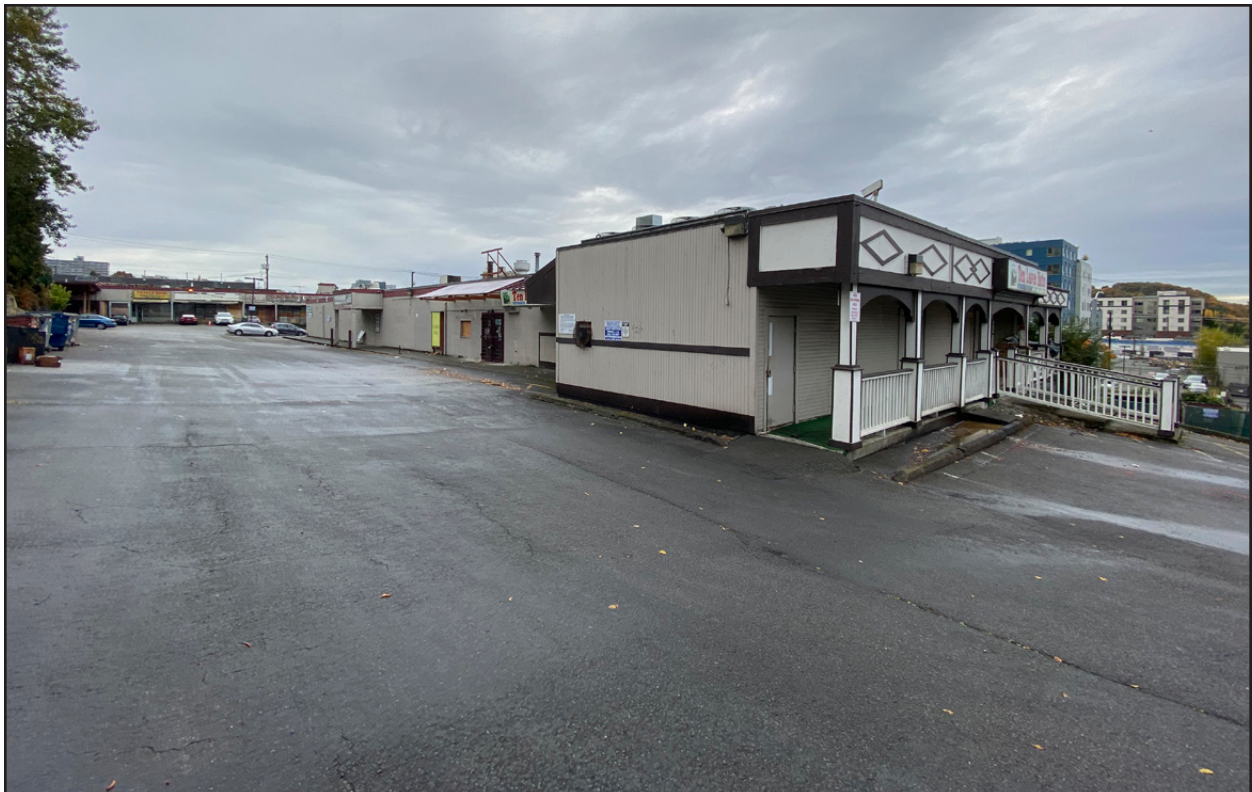
Figure 18 • Building 1, northern facade, viewing southeast
