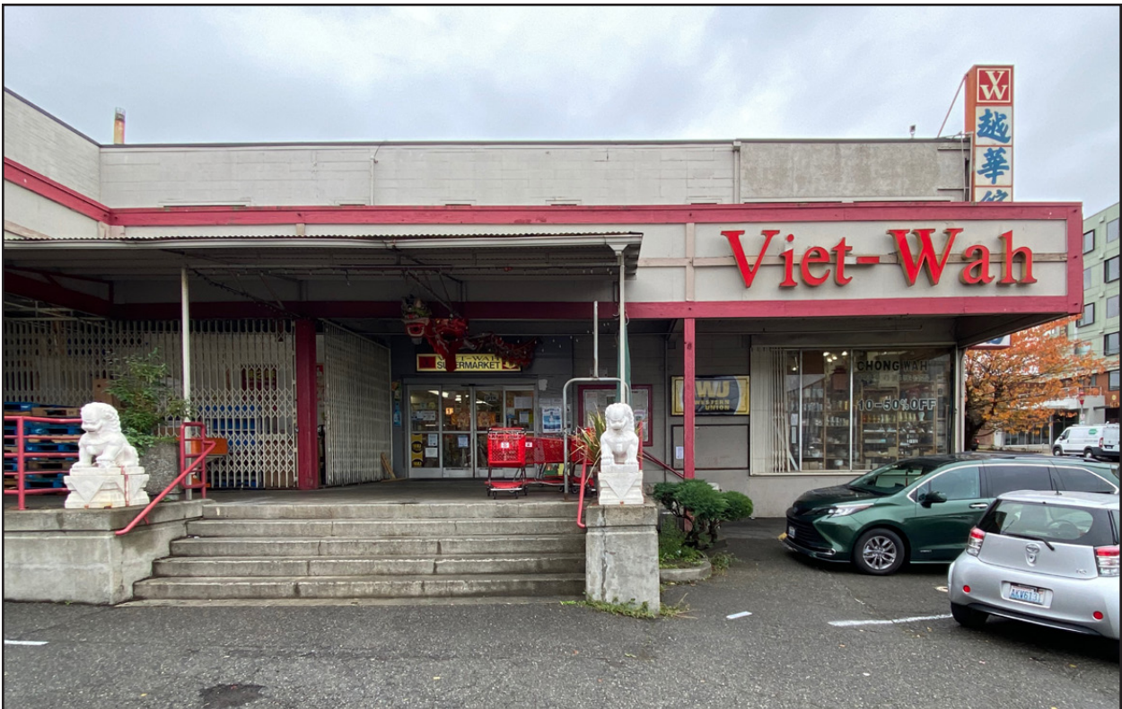
Figure 13 • Building 1, eastern facade and entry
