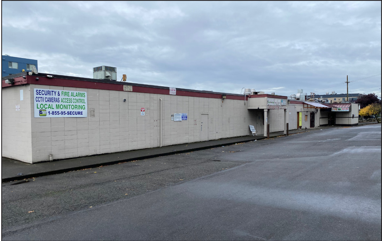
Figure 19 • building 1 northern facade, viewing southwest
