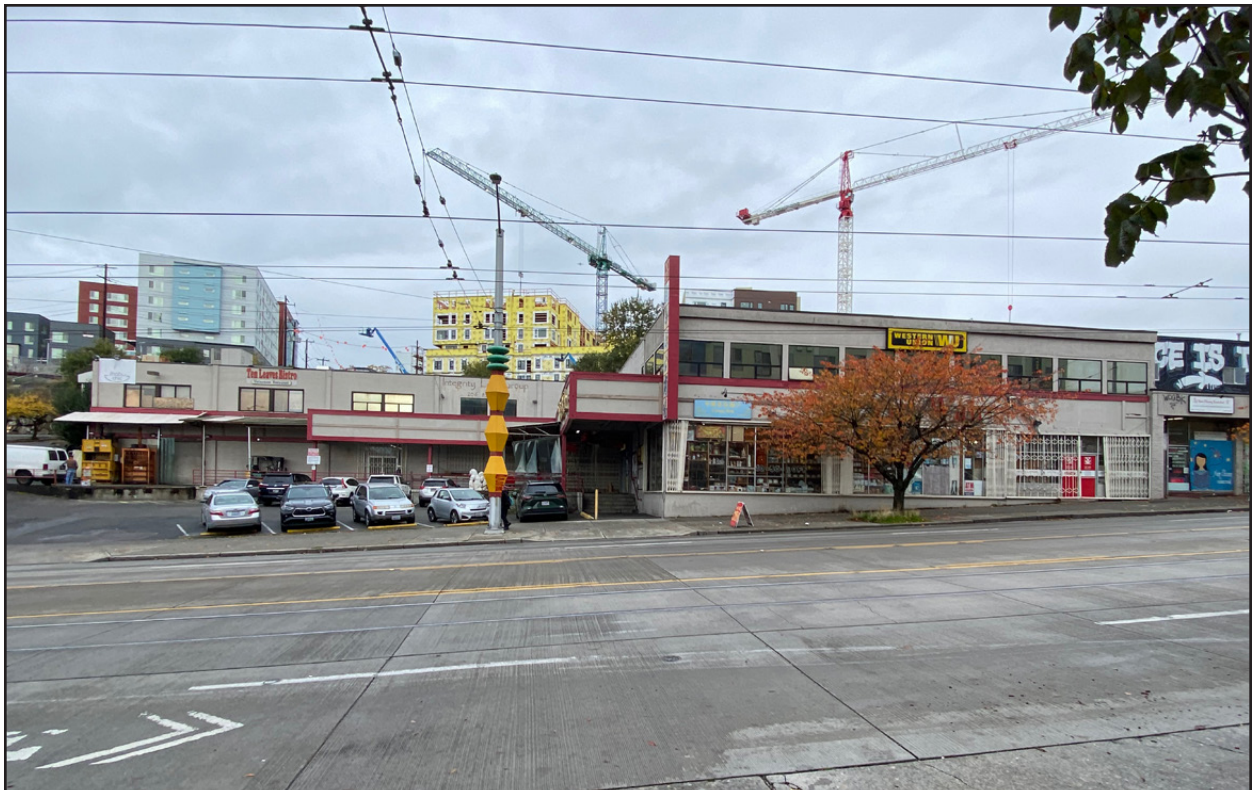
Figure 11 • Building 1 southern facade
