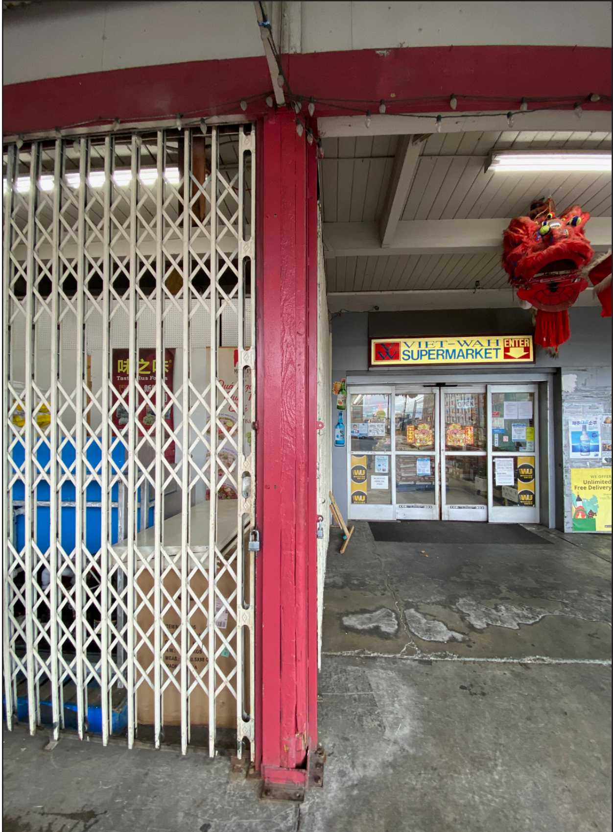
Figure 16 • Entry to building 1 at western facade.
