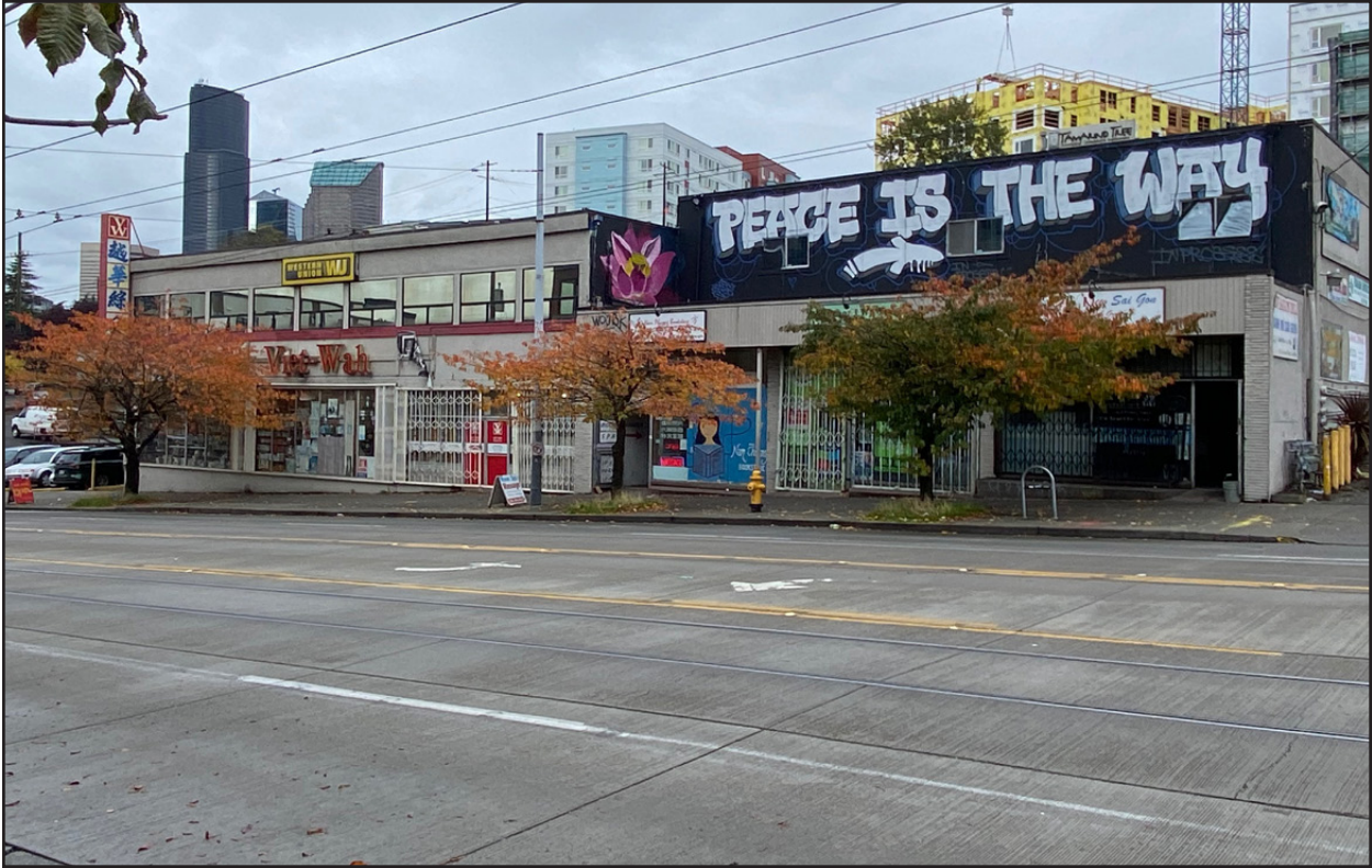
Figure 12 • Southern facades of building 1 and building 2
