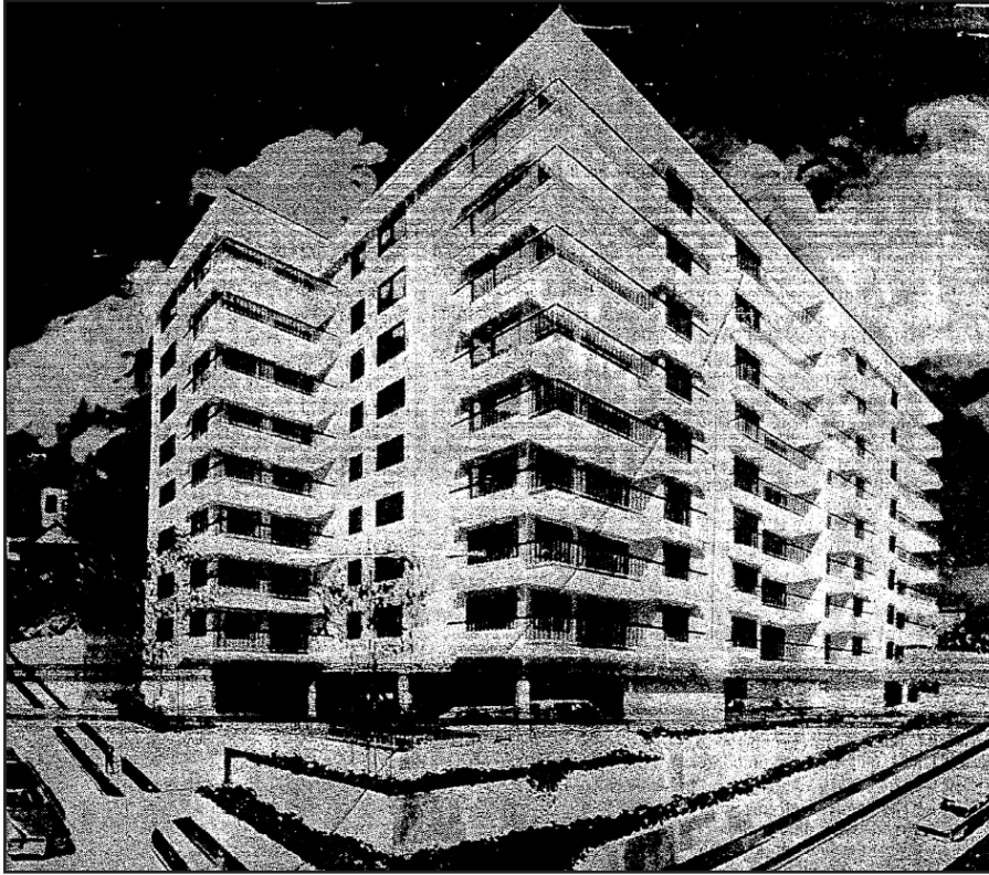
Figure 55 • Continental House, 100 Ward Street (1969, John Y. Sato & Associates, extant)
