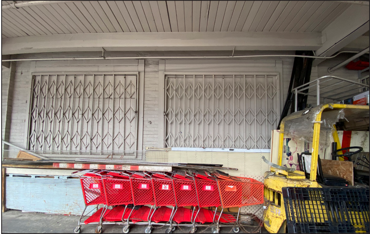
Figure 14 • Non-original boarded up openings at loading dock, building 1
