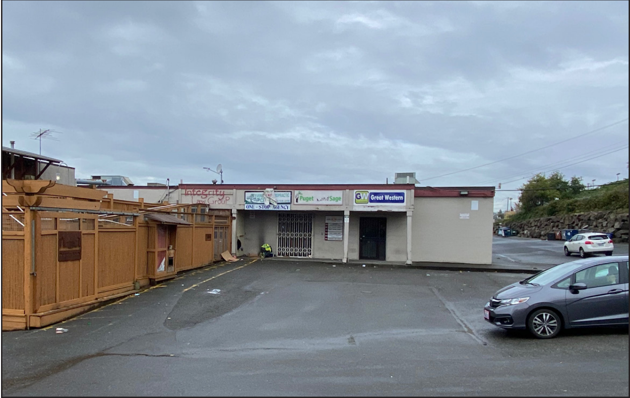
Figure 21 • Building 1, eastern facade
