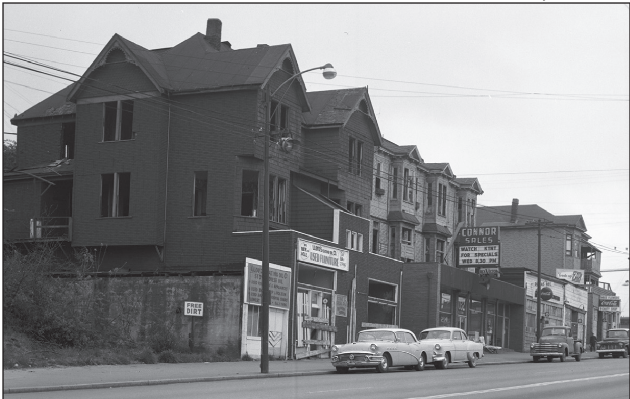
Figure 36 • North side of Jackson Street between 10th and 12th, before demolition.
