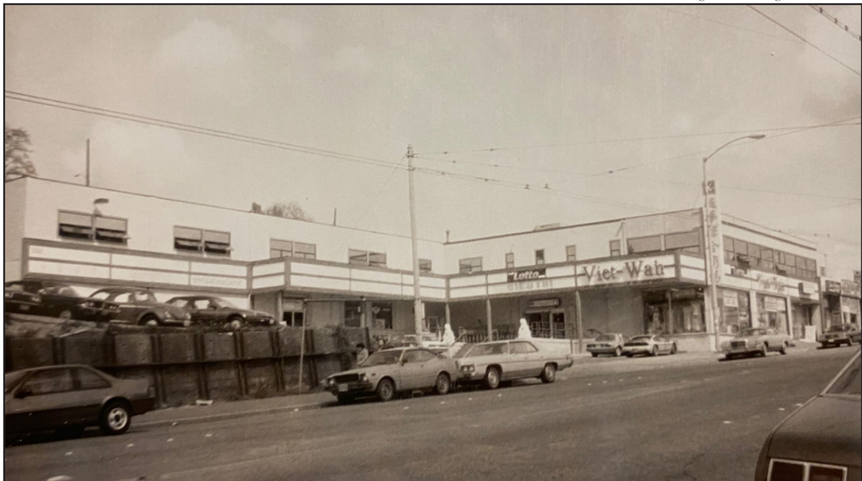
Figure 42 • Tax Assessor photo of subject building, ca. 1985
