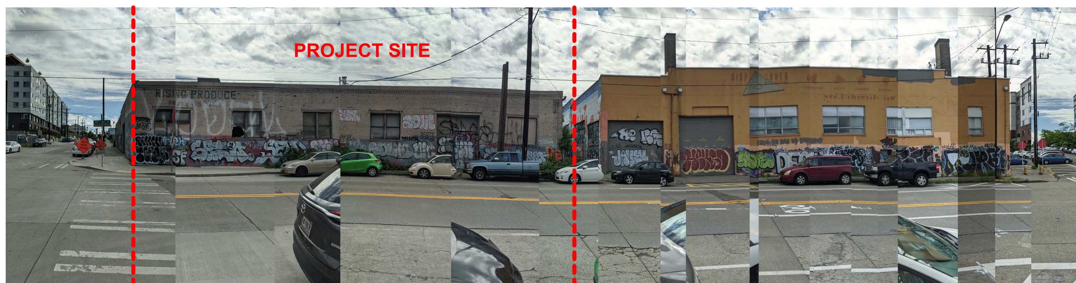
D - STREETScape ALONG 10th Ave. S TOWARDS EAST
