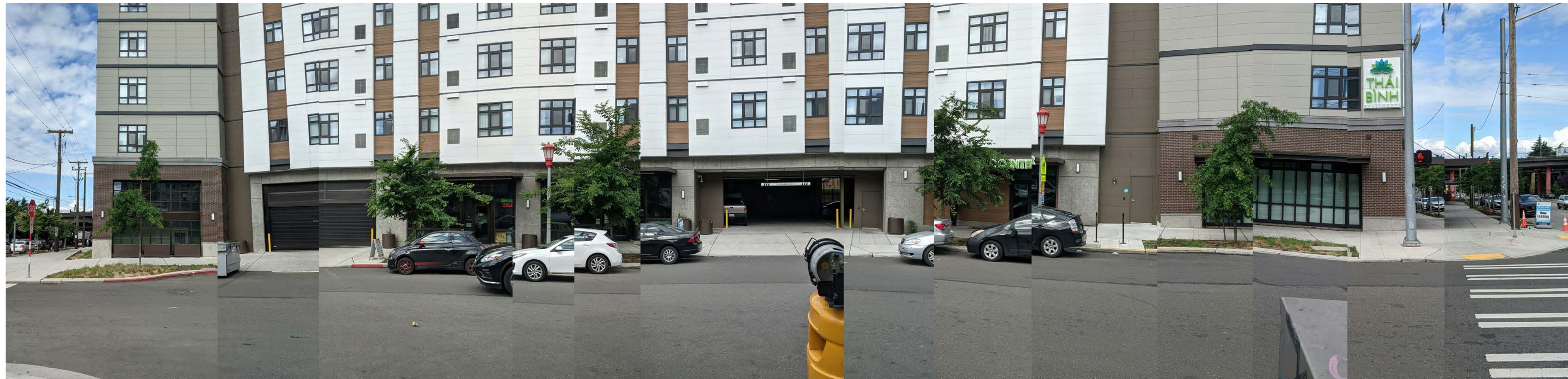
B - STREETScape ALONG 10th Ave. S TOWARDS WEST
