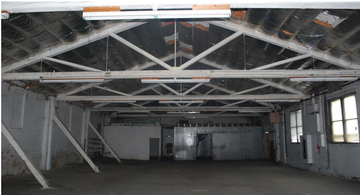
FIGURE 3.4a: 1001 S. King Street Interior Photo (Oct. 2018)
