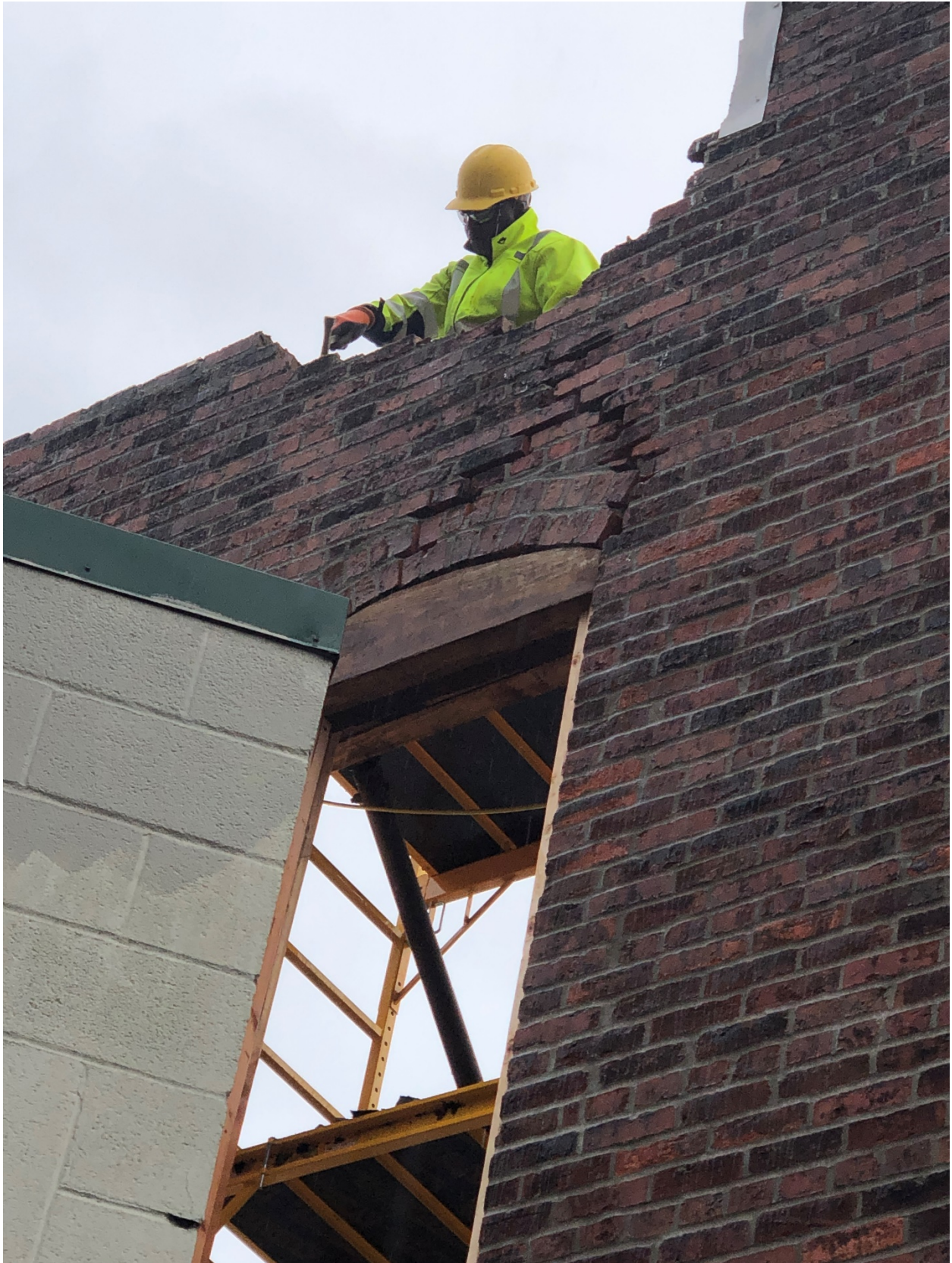
Masonry repairs and tuck pointing in progress.
