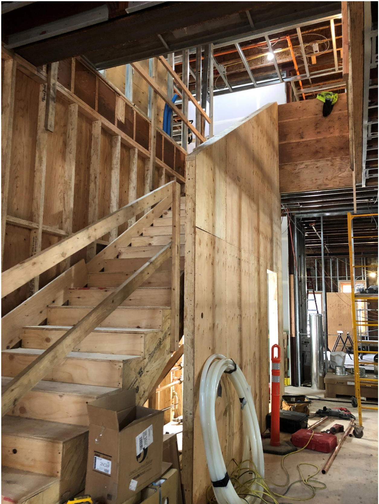
Framing new interior stair.
