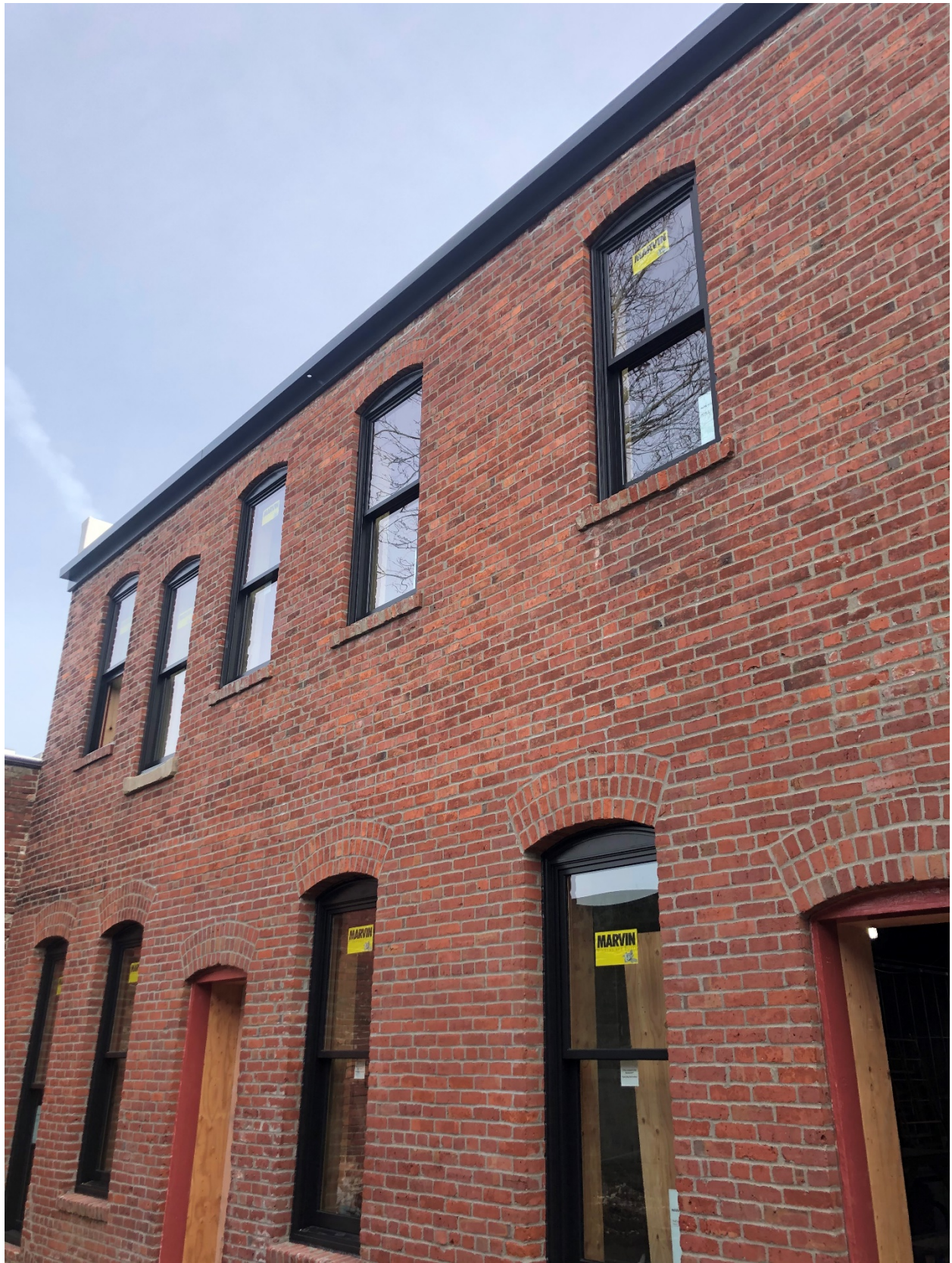
Exterior rear wall after tuck pointing and new window installation.
