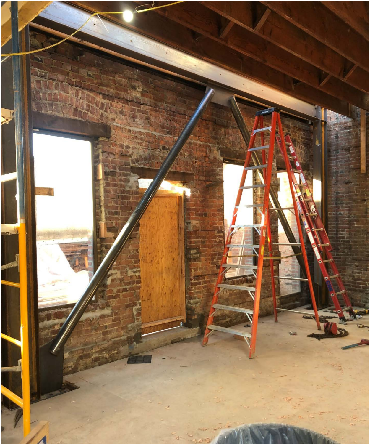
New 1 st floor seismic brace frame.
