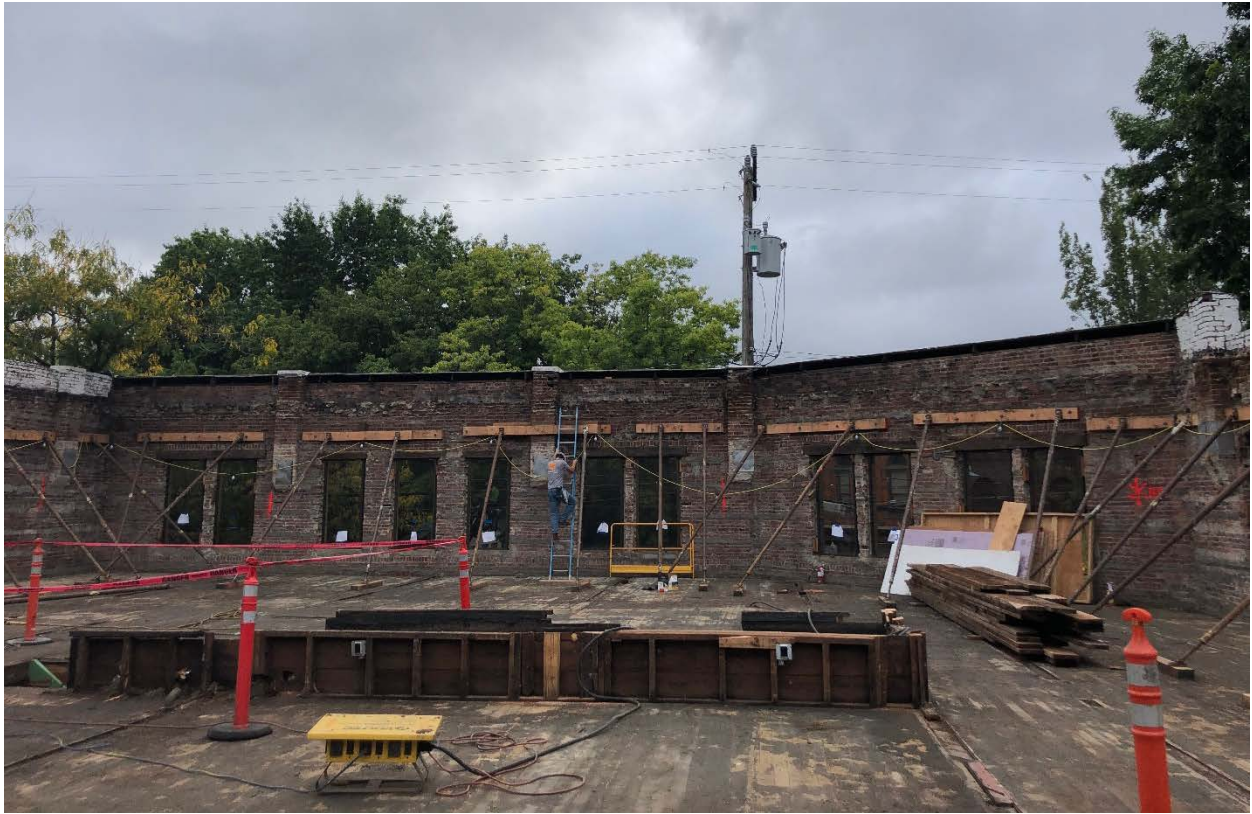
Roof structure completely removed and walls braced.
