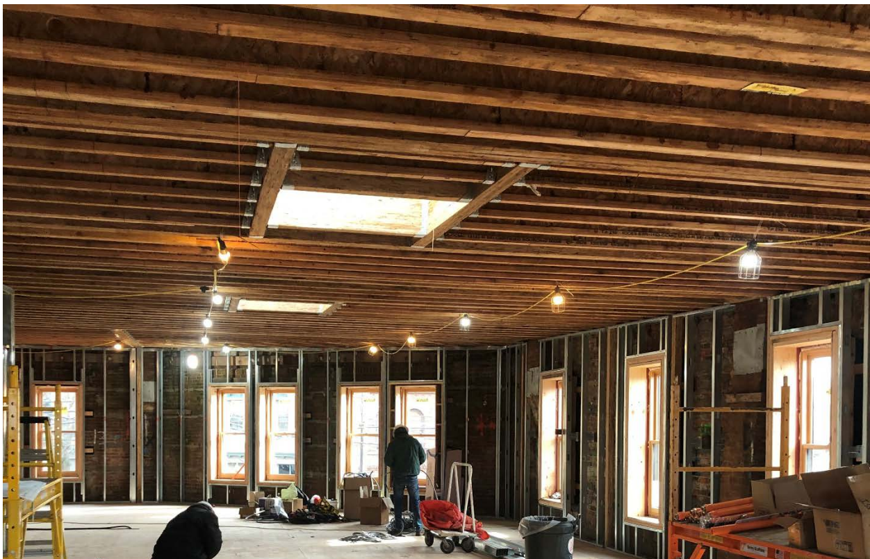
New roof structure and 2 nd floor interior wall framing with new windows and skylights.
