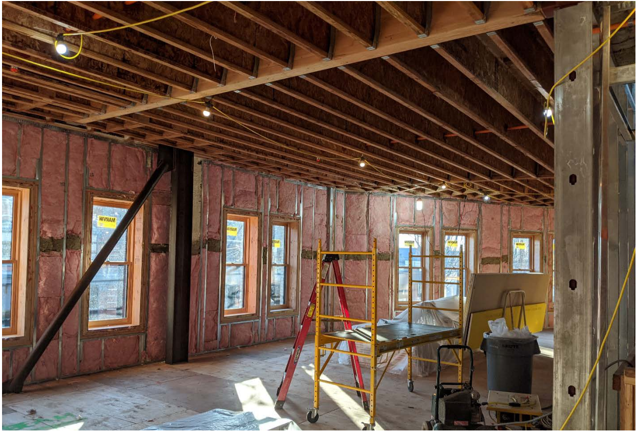
New 2 nd floor framing, seismic brace frame and insulation.
