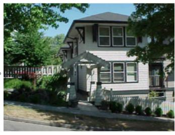
Broad roof eaves improve aesthetics, reduce thermal gain in summer and divert rain away from foundation.
