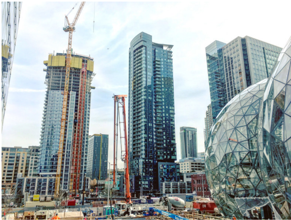
Construction in the Denny Triangle neighborhood of downtown Seattle, by Dan Bertolet, used with permission.
