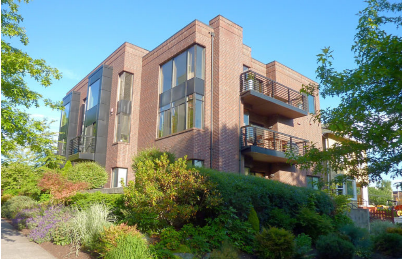
Three-story condo building at 16th and Pike in Seattle, by Dan Bertolet, used with permission.
