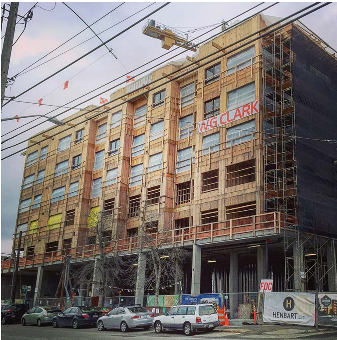
Typical “5-over-1” apartment construction with five stories of wood-frame on top of a concrete base, by Dan Bertolet (Used with permission.)
