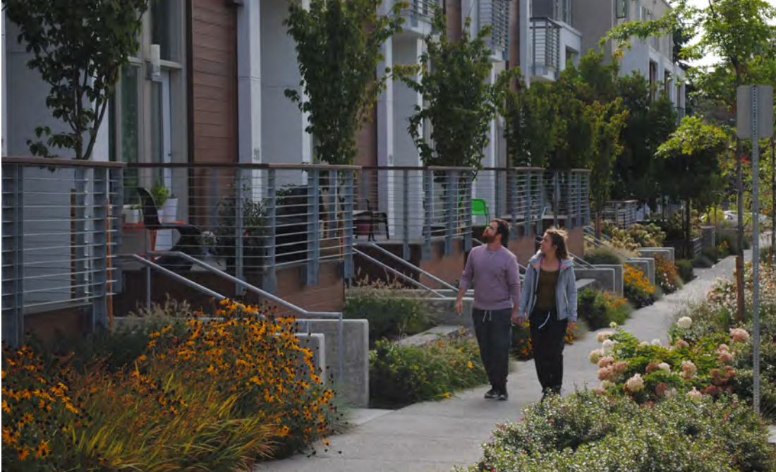
Urban design standards are proposed for privacy and design interest to address the edges of Lowrise zones.
