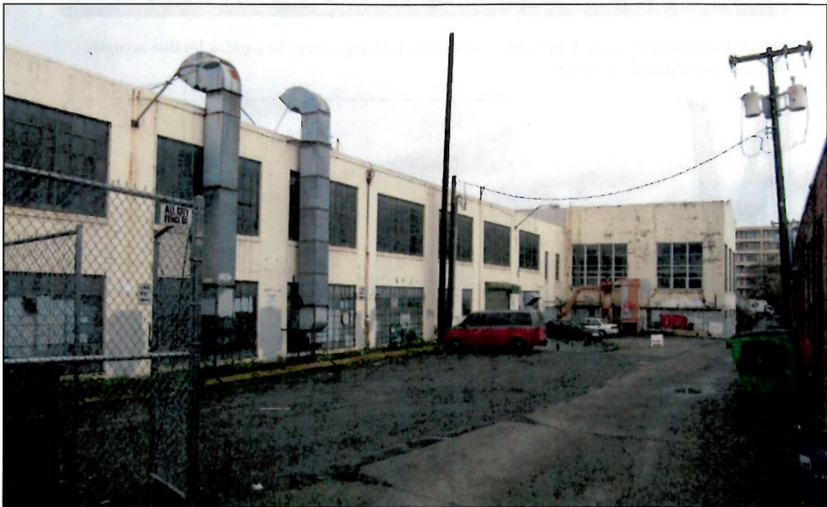
Figs. 31 and 32 Views of the east facade along the alley—top, view looking south; above, view looking north. The basement is at grade level on this side. Most original industrial steel sash windows are extant on this side of the building. Some newer aluminum framed windows have been inserted into original openings on the building's north and south wings.
