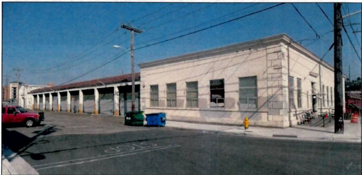
Figs. 18 and 19 Views of the primary west facade along 8th Avenue North—top, view looking southeast, showing the north end; above, view looking northeast. The series of columns and large openings of the clay tile-roofed central section gives the effect of an arcade set between the tall, gabled north wing and the flat-roofed south wing.
