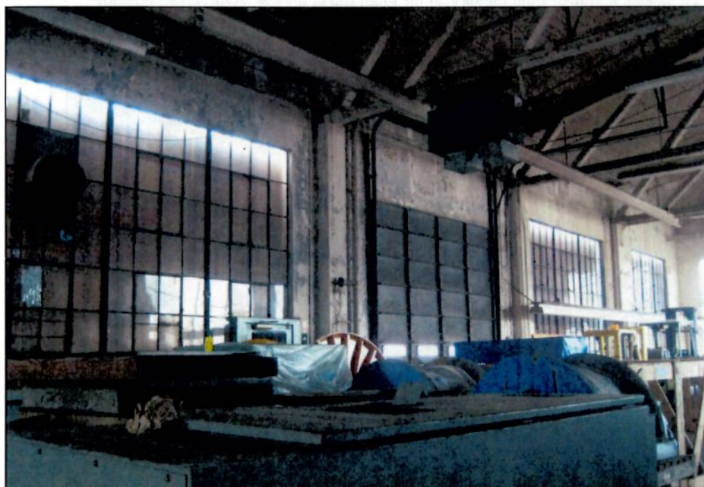
Figs. 35 and 36 Interior views in the north end of the building show the concrete frame, heavy timber trusses and car decking at the roof, the hoist way, and the typical large openings with industrial steel sash windows.
