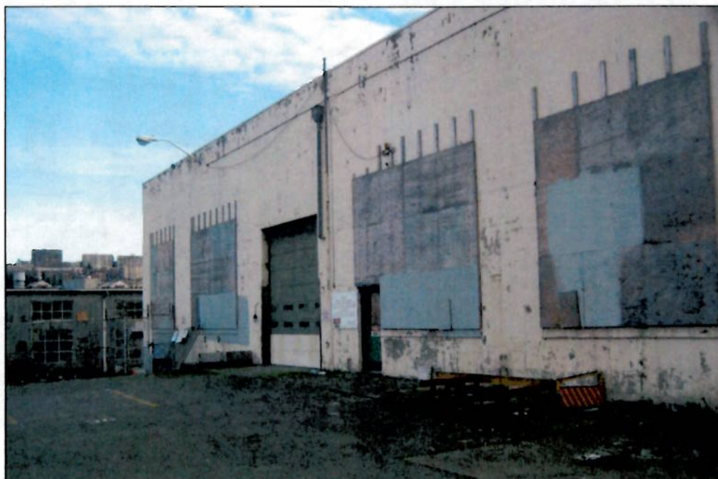
Fig. 28 Oblique view of the north facade. Original multi-light steel industrial sash windows remain in place behind the protective plywood covering.
