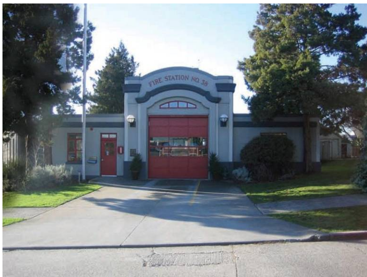
Former Fire Station looking east from 33 rd Avenue NE
