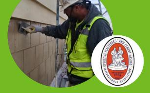
use conventional plaster, veneer plaster, stucco, weather barriers, exterior insulated finish systems, fireproofing and more products. Must be in physical shape and have good balance, eyesight and hearing. Plasterers work indoors and out. They are required to work from heights on scaffolding, swing stage and lifts.
