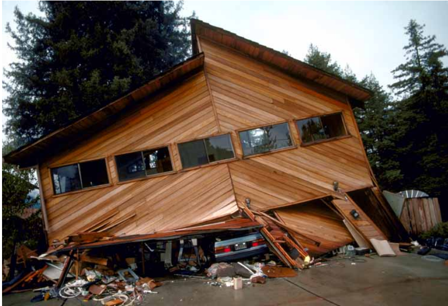
Figure 5-8. Home Damage Due to Inadequate Cripple Walls
