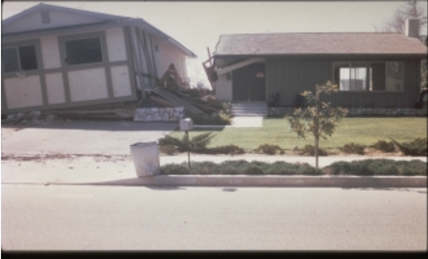
Figure 5. Collapse of garage. The large garage door opening weakens the ability of the structure to resist earthquake shaking (Photo from Applied Technology Council)
