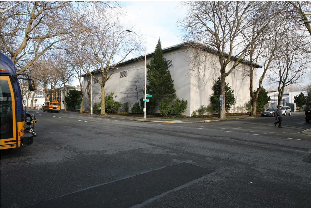
Photograph 26: 2017 view of the southwest corner of the NASA Building. Courtesy Artifacts Consulting, Inc.
