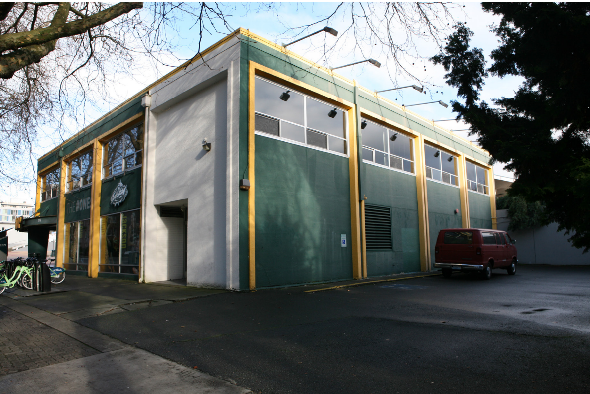
Photograph 34: 2017 view of the southwest corner of the West Court Building. Courtesy Artifacts Consulting, Inc.
