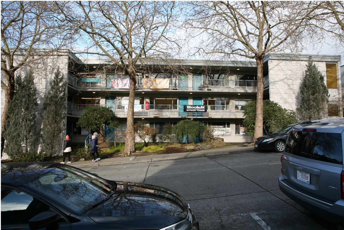
Photograph 37: 2017 view of the south elevation of the Blue Spruce Building. Courtesy Artifacts Consulting, Inc.
