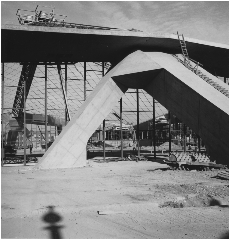
Photograph 21: Coliseum construction photograph. Courtesy Seattle Municipal Archives, #167425.
