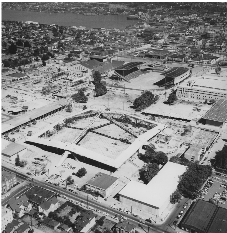
Photograph 2: Coliseum construction, November 1961. Courtesy Seattle Municipal Archives, #167458.
