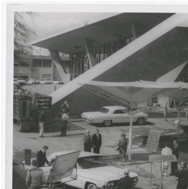
Photograph 8: View of the Coliseum in 1962. Note the absence of downspouts. Courtesy Seattle Public Library, Century 21 Exposition digital collection.
