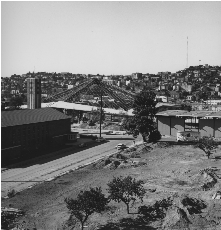
Photograph 4: Coliseum construction, 1961. Courtesy Seattle Municipal Archives, #167426.
