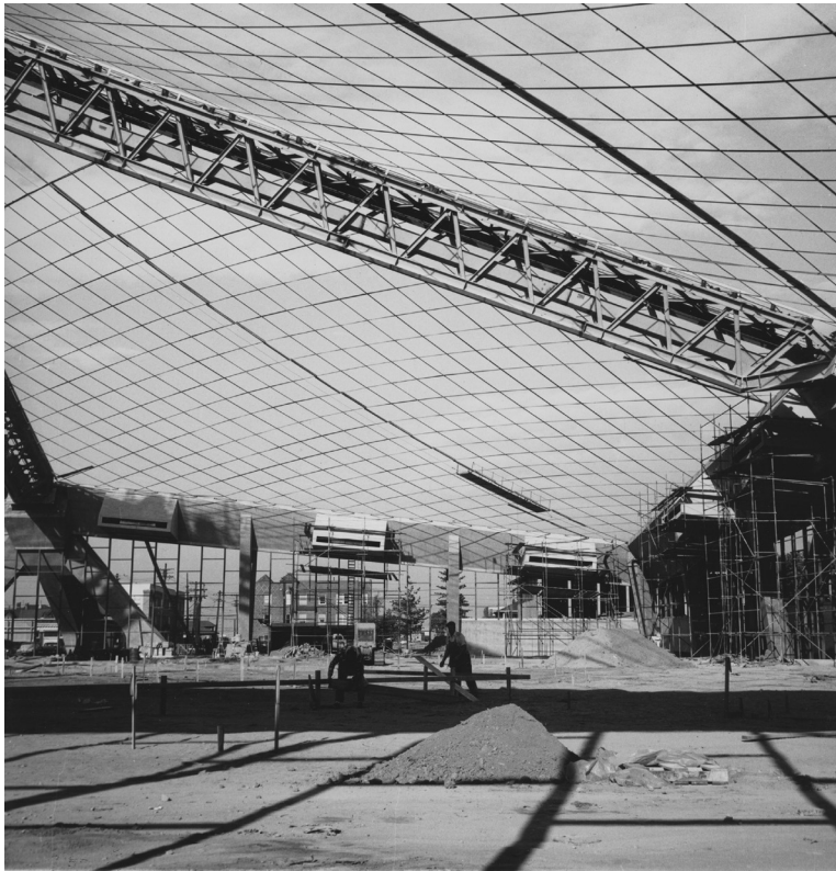
Photograph 3: Coliseum construction, 1961. Courtesy Seattle Municipal Archives, #167424.
