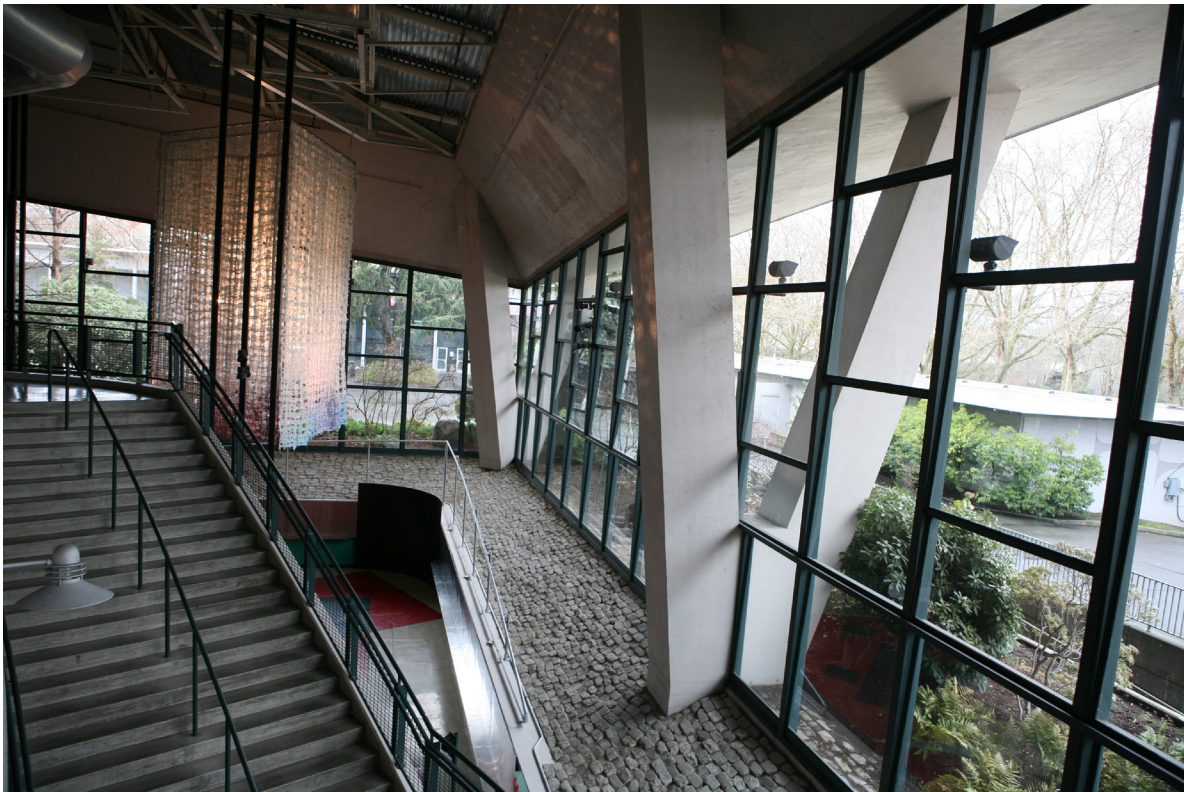
Photograph 46: 2017 interior view of KeyArena, showing glass curtain wall, concrete supports, and cobblestones. Courtesy Artifacts Consulting, Inc.
