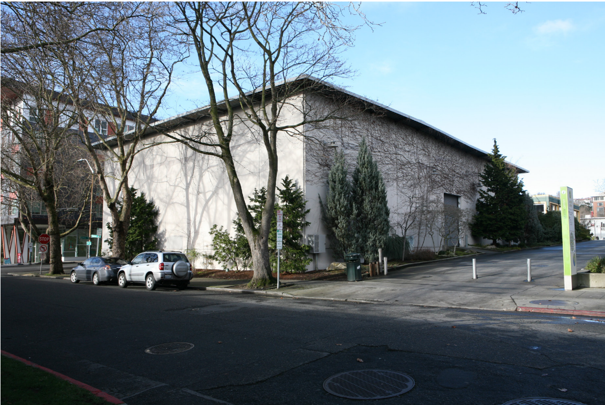
Photograph 29: 2017 view of the southeast corner of the NASA Building. Courtesy Artifacts Consulting, Inc.
