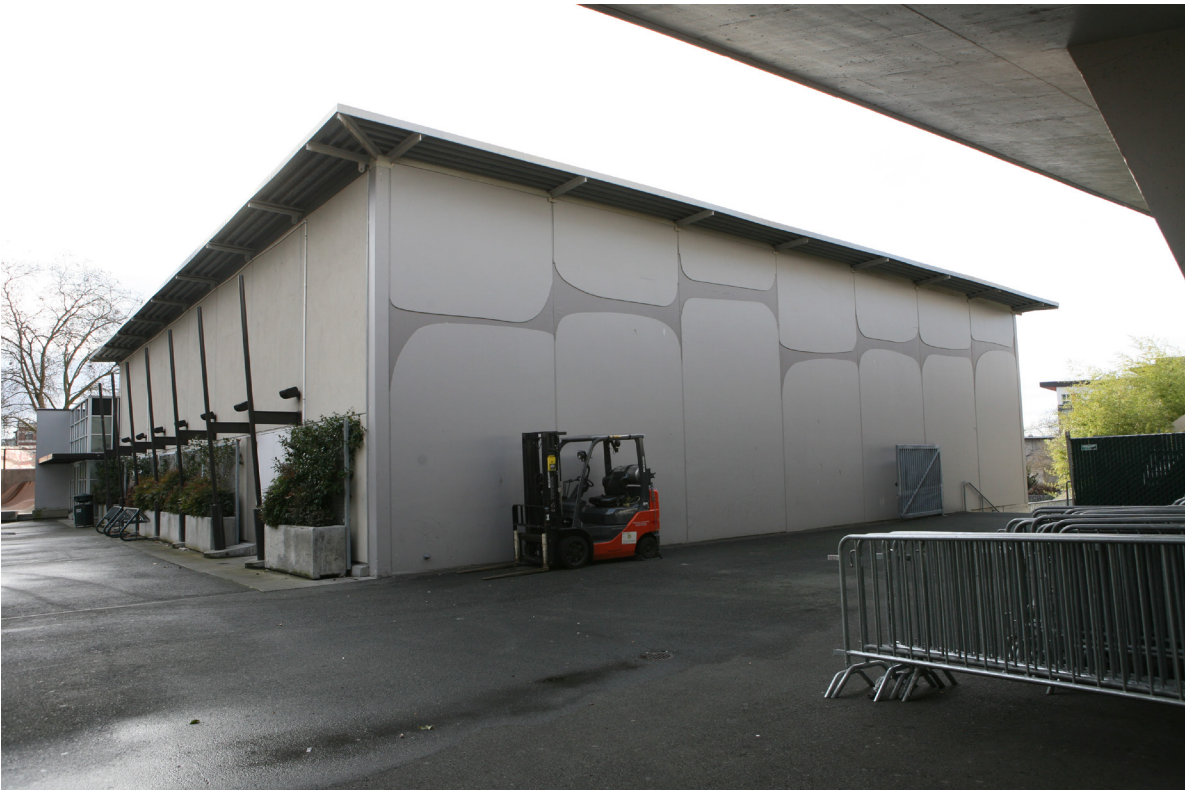
Photograph 42: 2017 view of the northeast corner of the Seattle Center Pavilion. Courtesy Artifacts Consulting, Inc.
