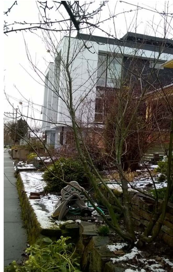
New Construction – no set back; overwhelms adjacent building.
