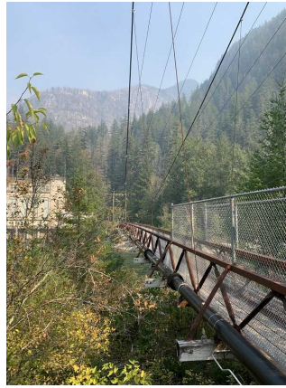
Transmission line conduit seen on south (right) side of Gorge Pedestrian Suspension Bridge.
