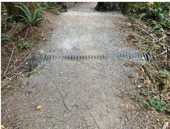
Trail of the Cedars gravel surfacing and plastic barrel culvert, facing east.
