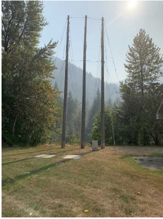
Transmission line northern bank pole triplet and overhead lines, facing south.
