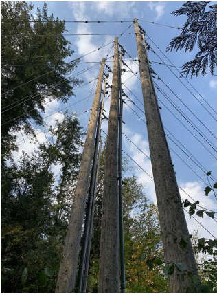
Transmission line detail view of vertical conduits on southern bank pole triplet and overhead lines, facing west.
