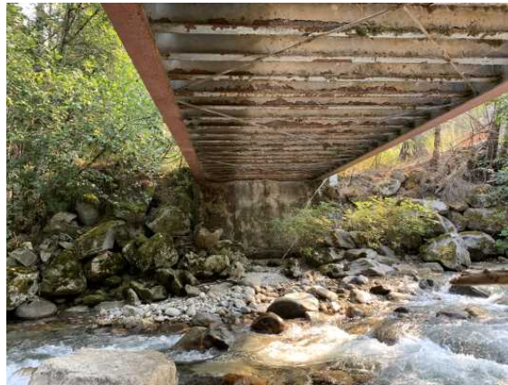
Underside of Newhalem Creek Bridge showing diagonal girder supports and east concrete abutment, facing east.
