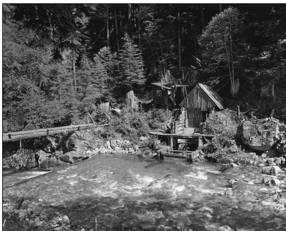
Figure 8. 1921 NCPDC headworks in 1949 with dam and log bridge at left and timber intake and gatehouse at right, facing east
