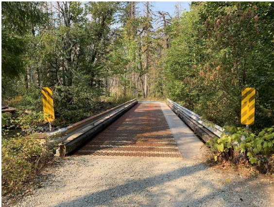
Newhalem Creek Bridge, showing metal grate deck and steel plate ADA deck alteration, facing west.
