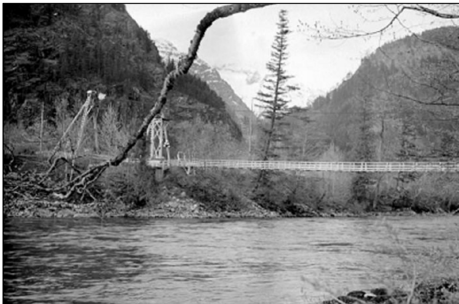
Figure 5. Skagit River cableway skidding system and traveler in 1937 with 1920 Newhalem Suspension Bridge in background, facing northeast
