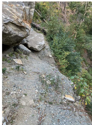
Dam Access Road at landslide, facing north. Detail metal netting for road surfacing retention exposed through landslide.
