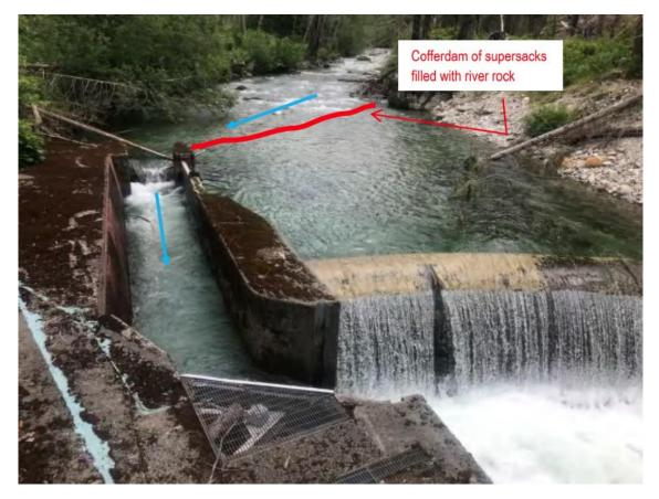
Figure 2. Water diversion structure including dam and impoundment and also showing location where cofferdam would be placed during dam removal. (Source: City Light, 2022a).
