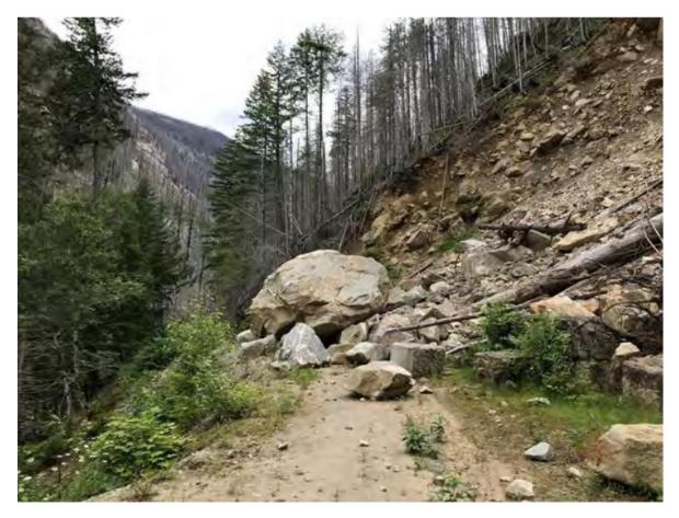
Figure 4. Rock slides along the dam access road. Older debris slide deposits are exposed in the right lateral scarp in the middle distance. (Source: City Light, 2022a).
