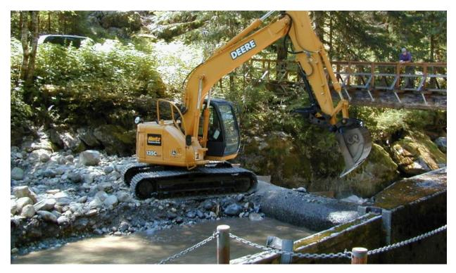
Figure 6. Annual excavation and downstream placement of accumulated sediment upstream of the diversion dam (year 2005) (Source: City Light, 2022d).
