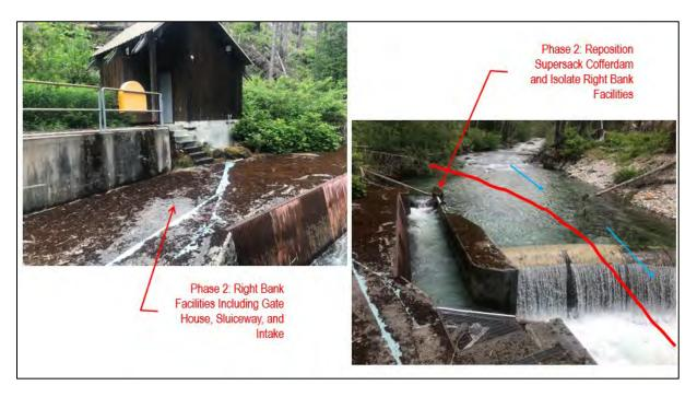
Figure 2.2-7. Right bank infrastructure to be removed during Phase 2.
