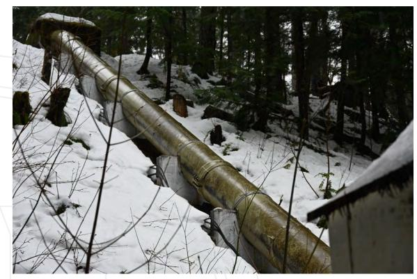
Figure 11. Final section of penstock from concrete thrust block to powerhouse, showing new concrete saddle supports, 2022.
