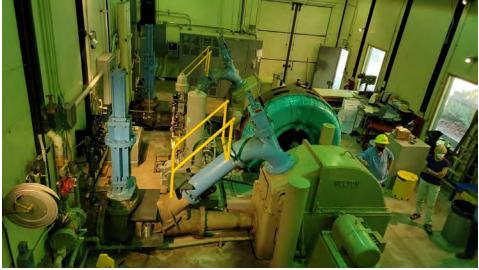
Figure A-4. Double Overhung Pelton Impulse Generator in Powerhouse
