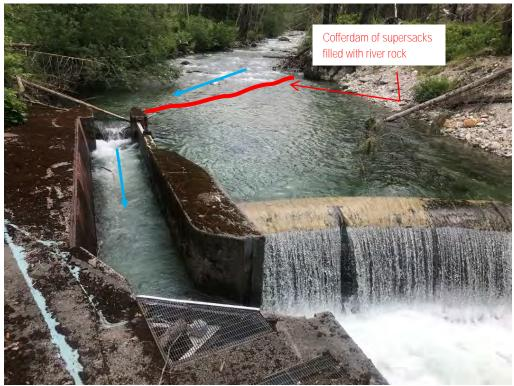
Figure E-1. Diagram of Phase 1 Supersack Placement and Water Diversion
