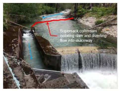
Figure 2.2-4. Phase 1 dam removal approach – divert creek into right bank sluiceway.
