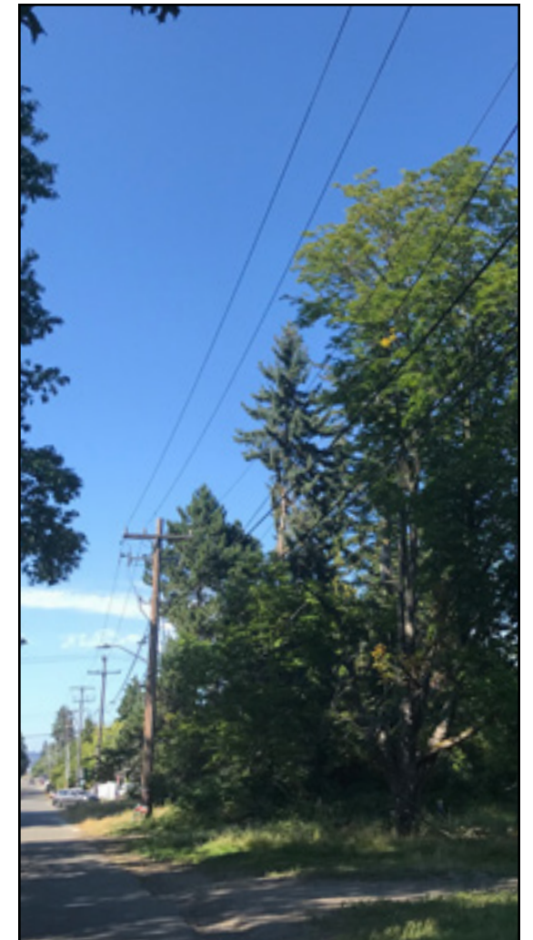
Delridge utility poles (photos: Vaughn Bell)
