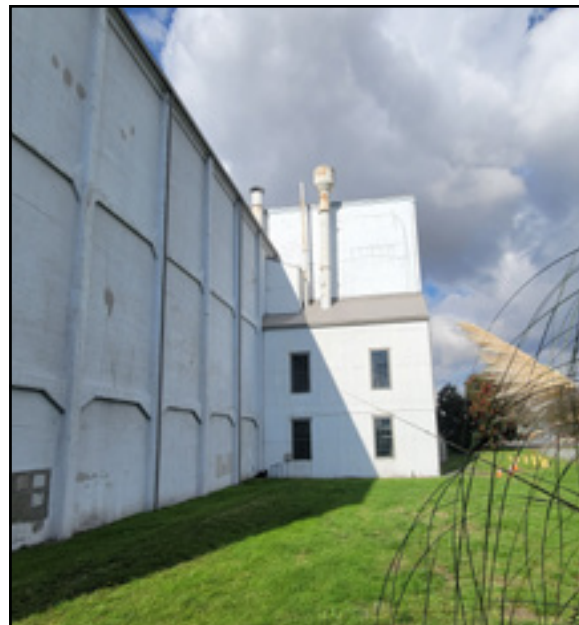
Exterior of Georgetown Steam Plant (photo: Kate Clark)
