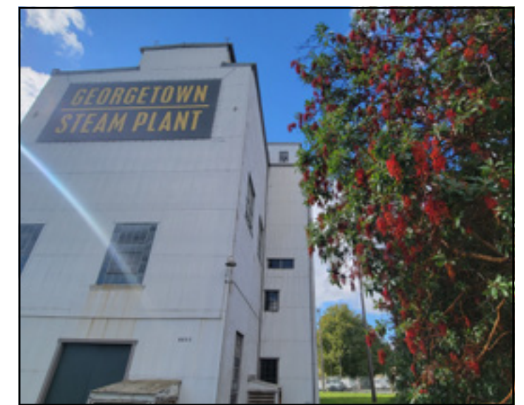
Georgetown Steam Plant [photos: Kate Clark]
