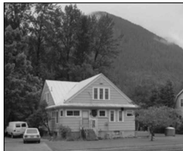
North facade, house no. 7, Silk Stocking Row, Newhalem, 1990. Skagit Power Development, Skagit River & Newhalem Creek Hydroelectric Project. Library of Congress, Photos from Survey HAER WA-24
