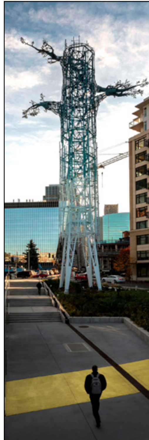
Lead Pencil Studio, Transforest , 2019. Seattle City Light Denny Substation.
