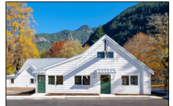
Gorge Inn Exterior Newhalem, WA. [photo: Basetti Architects]
