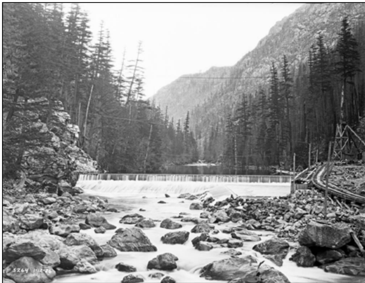
City Light's Gorge Dam intake on the Skagit River, with railroad on right, 1926. Courtesy Seattle Municipal Archives [2191]
