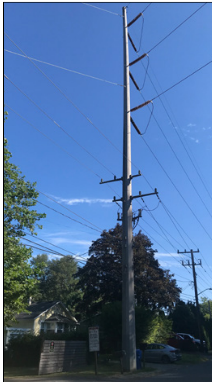
Delridge utility poles (photos: Vaughn Bell)
