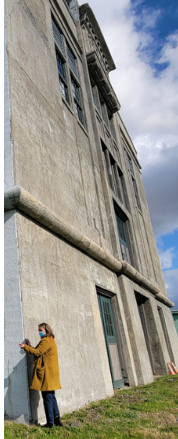
Georgetown Steam Plant tour with Senior Community Program Developer Julianna Ross
