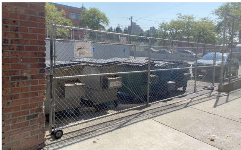
Figure 18: Canton alley owners secure dumpsters to deter illegal dumping and scavenging. Chain link fence is a CPTED-compliant option as it provides an open view into the trash enclosure for monitoring and safe access.
