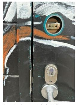
Image: Broken remote lock at Alki restroom.
