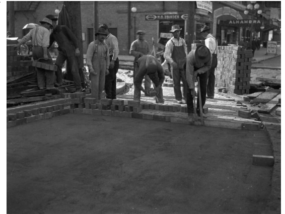
Workers laying brick for Pine St. paving, 1913. Item 6506 , Record Series 2613-07, SMA.
