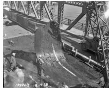
58063 Spokane Street Bridge #2. Redecking. [West Seattle Bridge]. August 14 1958
