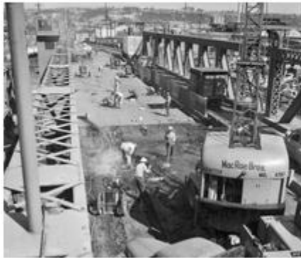
58061 Spokane Street Bridge #2. Redecking. [West Seattle Bridge]. August 14 1958
