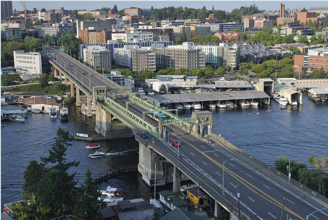
The University Bridge that connects the U District and Eastlake in District 4 was among the bridges ranked in “poor” condition along with the Magnolia Bridge, 2nd Avenue South extension, and the Fairview Avenue Bridge (which is being reconstructed). Photo: by SounderBruce on Wikipedia
