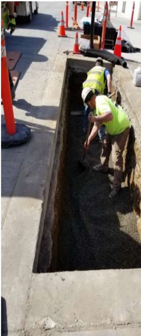
Place bedding and overflow infiltration stone layer
