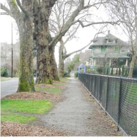
Decomposed granite, or small crushed gravel, may be used as a path / walkway surface in residential areas. It may also be used as a finished surface on top of planting soil in tree pits in areas of high pedestrian traffic (see 'Mulch').
