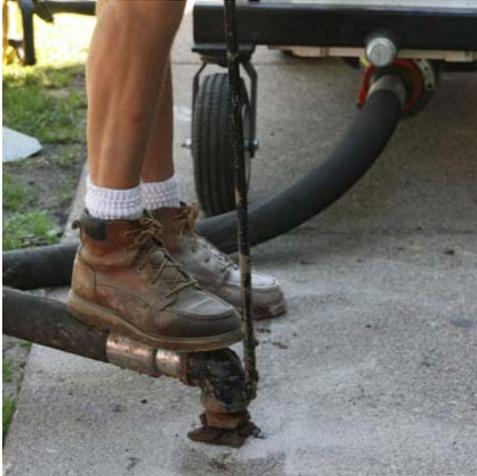
Mudjacking, or concrete leveling, is used to lift concrete panels when they have sunk or collapsed. Usually a cement and soil mixture is pumped under pressure below the existing concrete panel; the practice may also be performed using a foam fill material. The mixture fills the void beneath the surface and adds additional support under the concrete panel.
