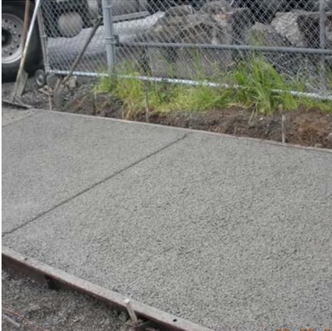
Pervious concrete allows air and water to pass through to the bedding and soil layers below. If designed and installed properly, it may deter shallow root growth (and reduce root damage to the sidewalk) by allowing water to infiltrate more deeply into the soil profile and providing air contact just below the pavement.
