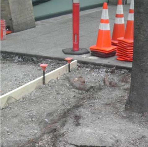
In some cases, thicker pavement may minimize future root damage by providing greater strength and resistance against root pressure. In other cases, thinner (reinforced) pavement can provide more space for existing tree roots.
