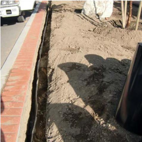
Root barriers are physical barriers (commonly plastic sheeting or interlocking panels) installed from surface level to a depth of 12”-24” or more at the interface between a tree zone and adjacent paving or other infrastructure. They are intended to deter root growth near the surface that may damage pavement. Typical placement is vertical, although horizontal root barriers also exist.
