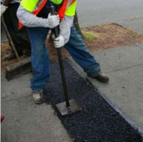
Shims, also called wedges, are temporary or interim measures to treat cracked or lifted sidewalks to reduce tripping hazards and improve accessibility. Asphalt is typically used to construct a shim.
