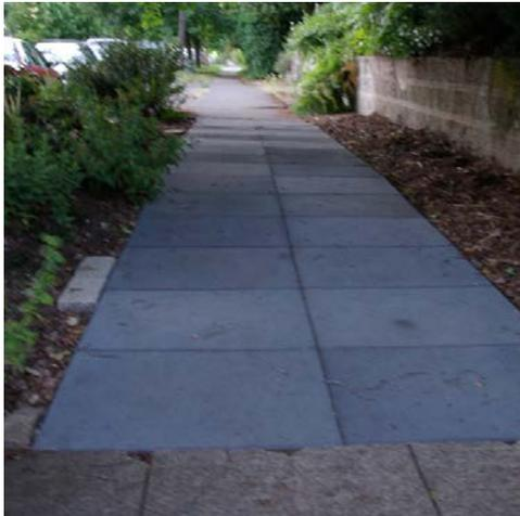
Many types of unit pavers are available, including several varieties made from materials such as rubber or composite plastics. When properly installed and maintained, pavers may provide accessible surfaces that are more flexible than concrete, providing room for continued tree root growth under the sidewalk.
