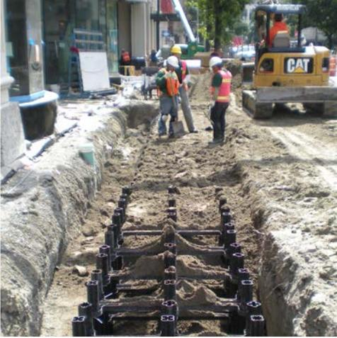
Suspended pavement systems may be used in new tree plantings where there is not an adequate volume of soil available for tree root growth. These systems provide structural support for pavement while allowing the use of planting soil as fill, which provides space for roots to grow, promoting healthy trees and preventing pavement damage by roots near the surface.
