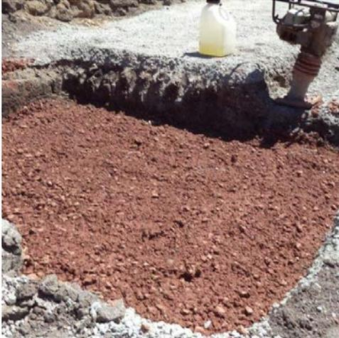
Structural soils are soils that are specially designed to provide nutrients, space, and porosity to accommodate root growth while also allowing for compaction to support pavement without settling. There are proprietary structural soil mixes available as well as various non-proprietary mixes that have been used in many municipalities.
