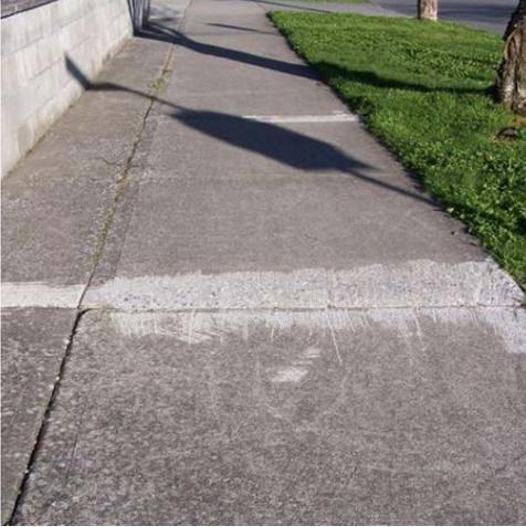
Beveling involves cutting down the raised edge of a concrete panel to make a smoother transition and reduce tripping hazards.
