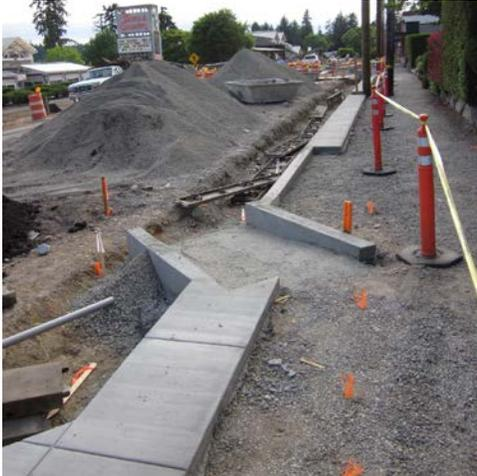
An open-graded gravel base course may be applied under the sidewalk pavement to discourage root growth directly under the pavement and reduce likelihood of sidewalk damage.
