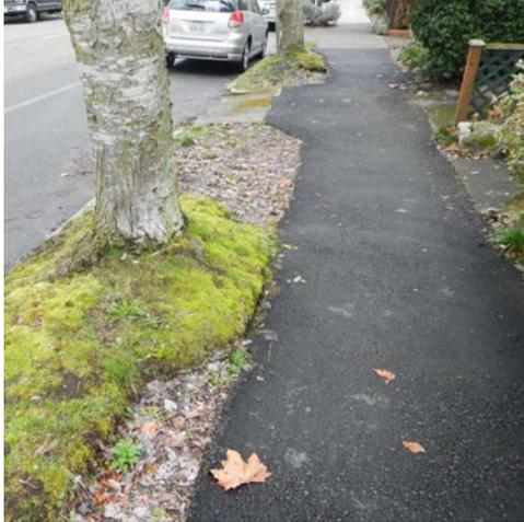
Asphalt is not typically used as a standard sidewalk material in Seattle; however, it may be used as a short- to medium-term pavement solution for sidewalk repair or replacement. It has less initial cost, is more flexible, and can more easily be repaired than concrete pavement. However, asphalt has a much shorter expected useful life and requires a higher level of ongoing maintenance than concrete.
