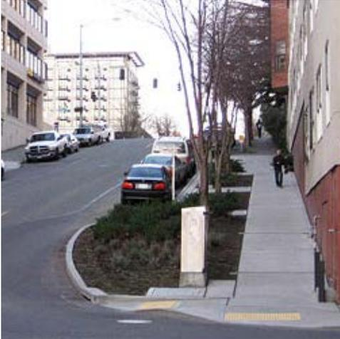
A curb bulb is a radial extension of a sidewalk at an intersection used to shorten the crossing distance for pedestrians. Curb bulbs may be landscaped and provide additional root growth area for trees, and can improve pedestrian crossings. Designs that include trees and landscaping must ensure proper sight lines are maintained.
