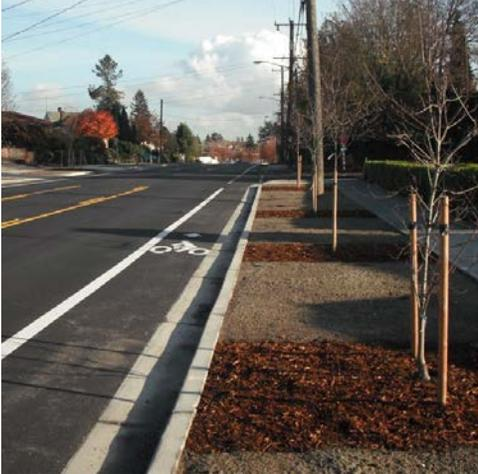
Curb realignment involves shifting the curb location for a significant distance (e.g., along an entire block) in order to widen the planting strip and provide more space for trees.
